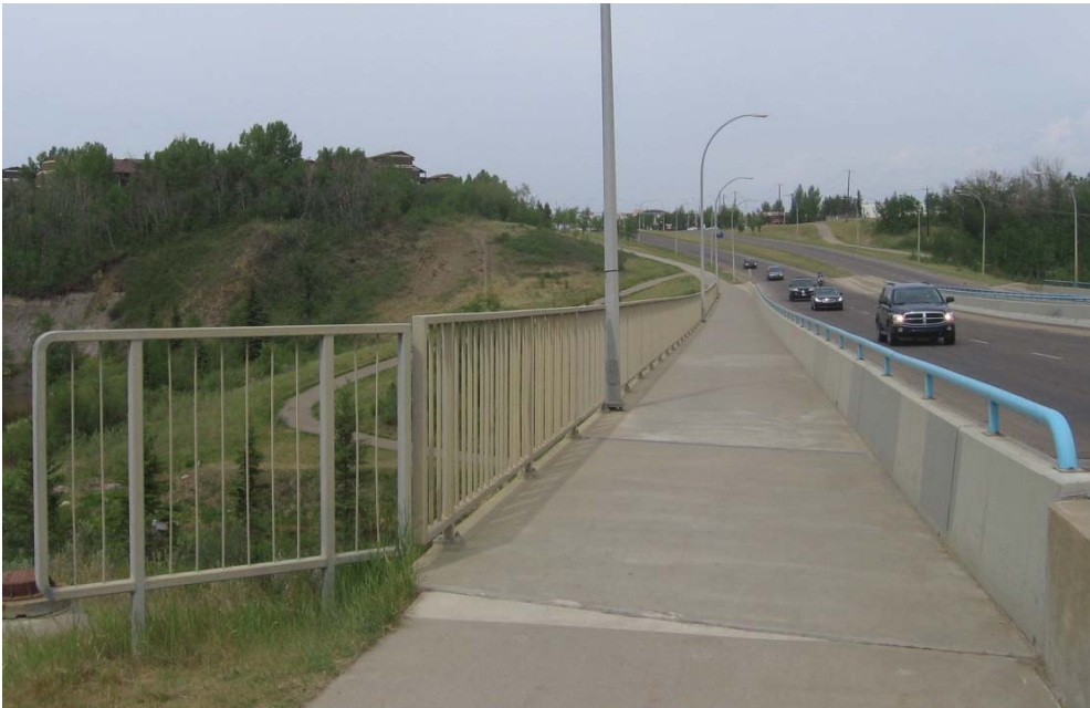
Existing Blackmud Creek Bridge Northbound
