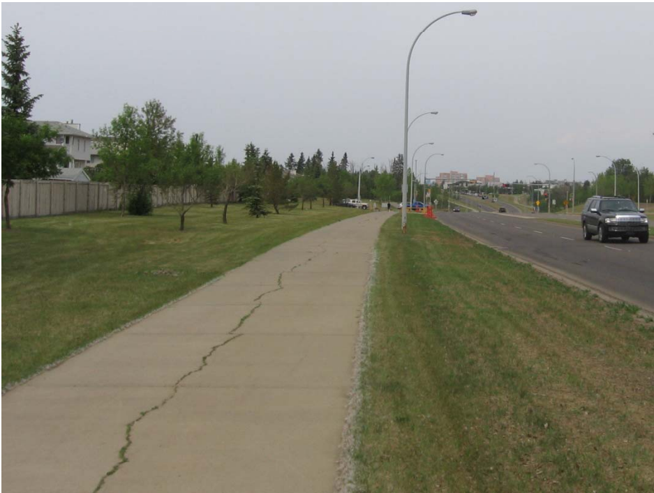
Existing 111 Street/ 9 Ave Northbound
