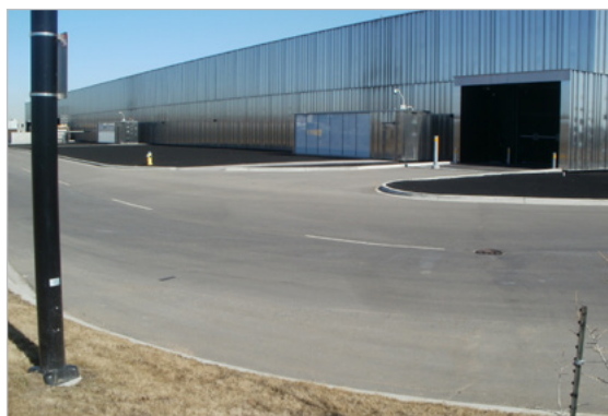
Grading of a Commercial property with slope and swale towards a catch basin within private property
