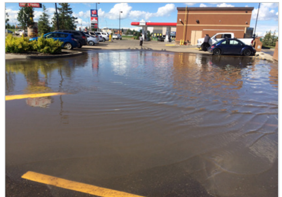
Stormwater is stored and drains slowly into a catch basin during and after storm events.
