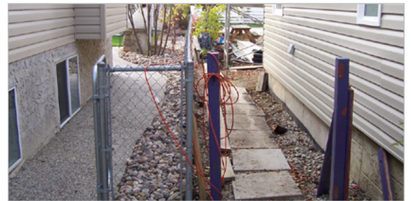
The new sidewalk on the left has the minimum 15 cm drainage space requirement within the property that drains surface runoff towards the street.
