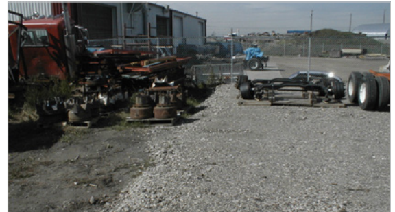
The new industrial development has no on-site stormwater management. The gravel is graded high and slopes towards the existing industrial site behind the fence.
