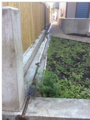
Concrete retaining wall and internal swale
