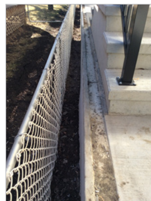
Concrete internal swale adjacent to concrete sidewalk
