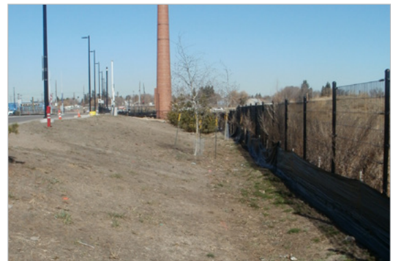
New commercial development with slope from an adjacent property into an internal swale
