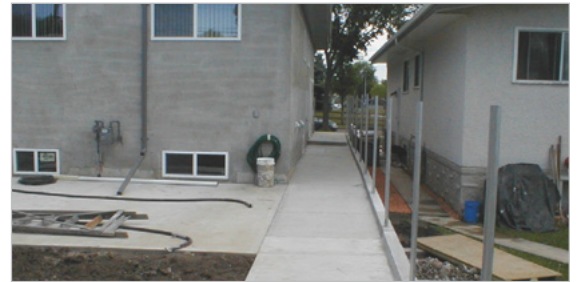
These new sidewalks with raised edges create internal swales that prevent surface water from draining towards the abutting lots.
