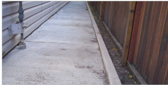
These new sidewalks with raised edges create internal swales that prevent surface water from draining towards the abutting lots.
