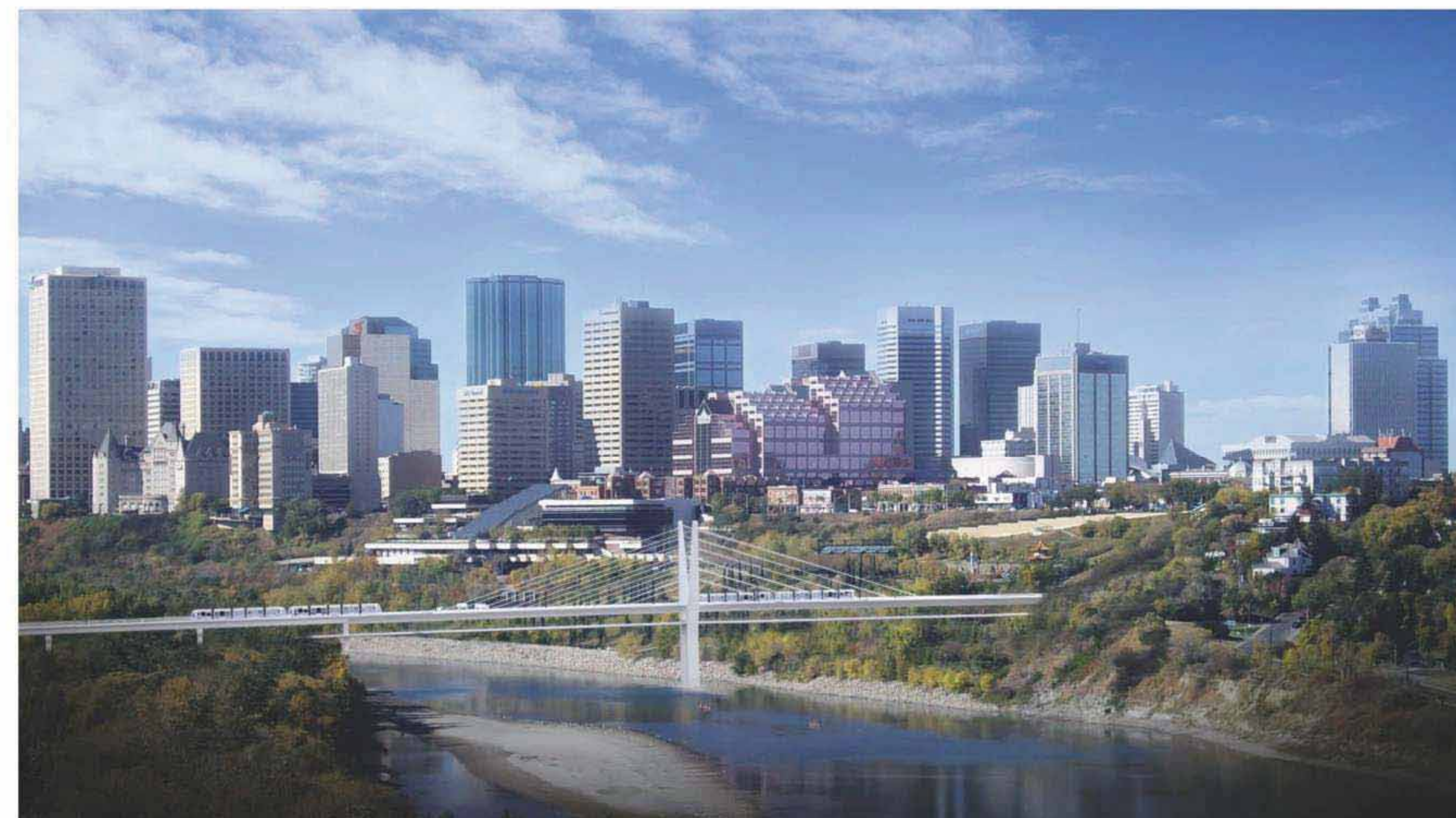
Option 2 - Extradosed bridge looking Northwest
