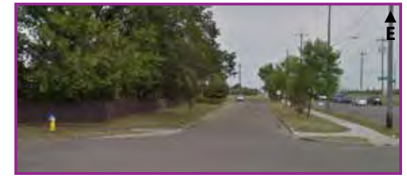
Missing sidewalk along the north side of the 127 Avenue service road between 113A Street and the alley west of 115 Street.
