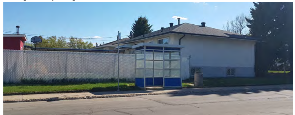
Existing Bus Stop Along 130 Avenue
