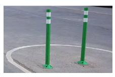
Figure 15. 36A Avenue – Example image of flexible bollards
