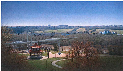
Extradosed bridge looking Southeast
