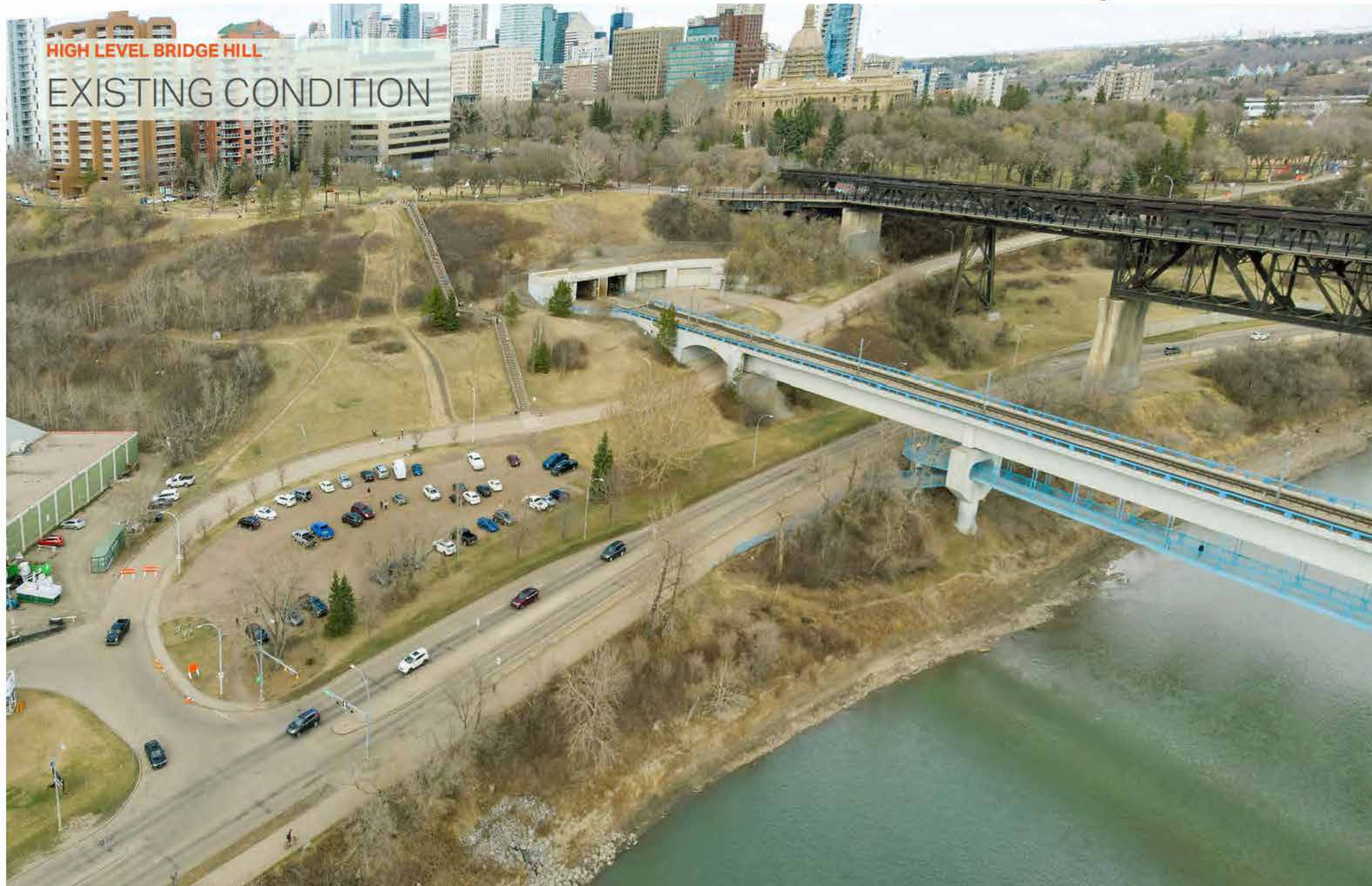
Figure 29. High Level Bridge Hill - Existing Conditions
