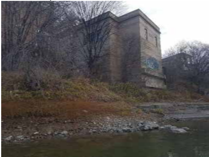
Plate 35: Looking at the downstream side of Pumphouse 1
