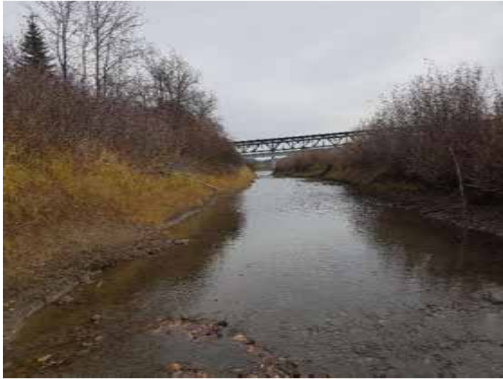
Plate 29: Looking downstream of the upstream end of the island side channel.
