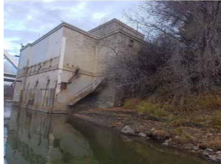
Plate 34: Looking at upstream at Pumphouse 2.
