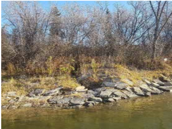
Plate 27: Looking at concrete riprap on the RUB between Transect 7 and Transect 8
