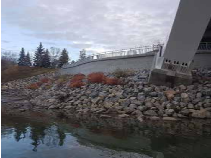
Plate 33: Looking at the Walterdale Bridge riprap at the downstream end of the Project Area.
