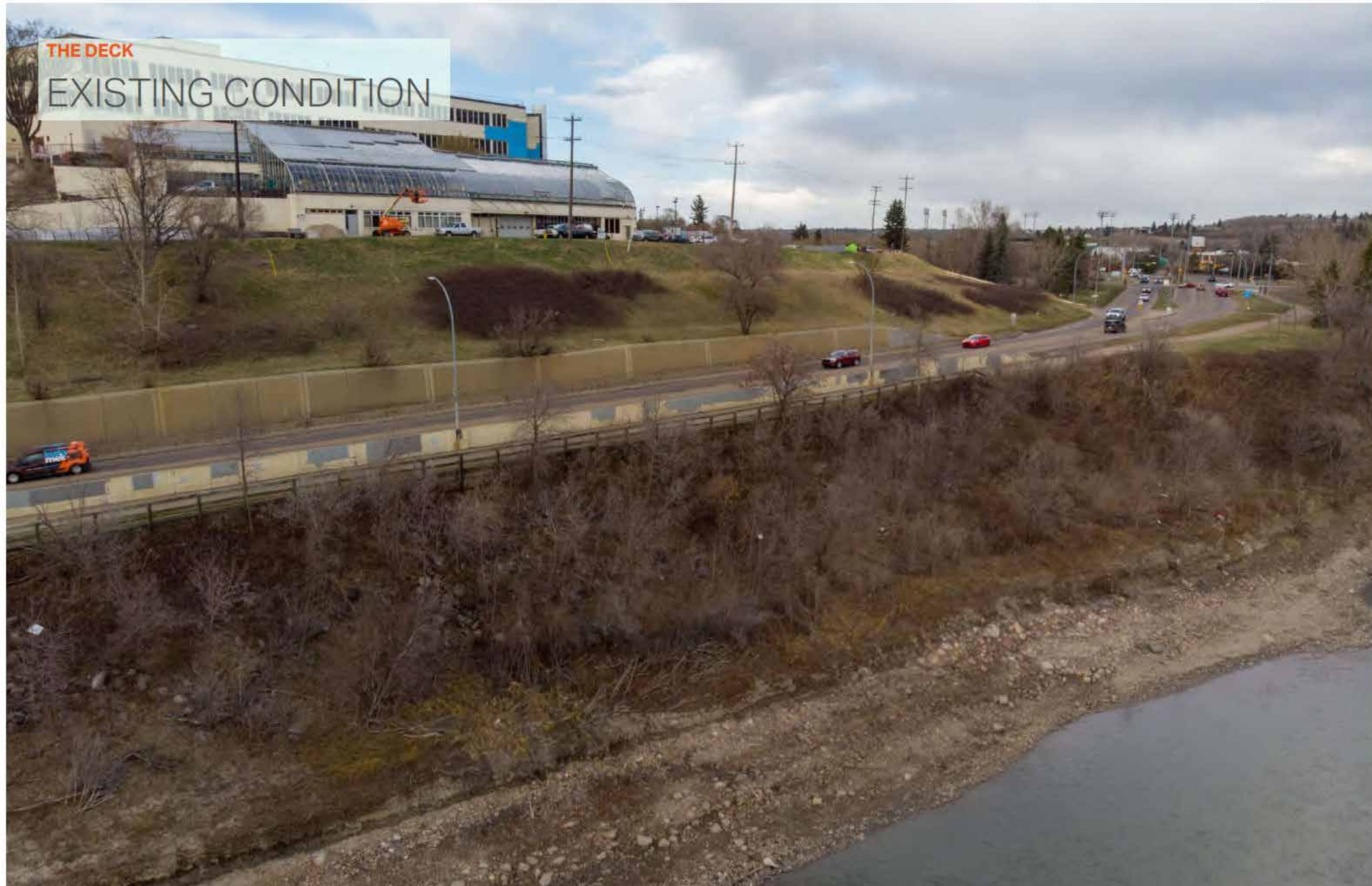
Figure 35. The Deck - Existing Conditions
