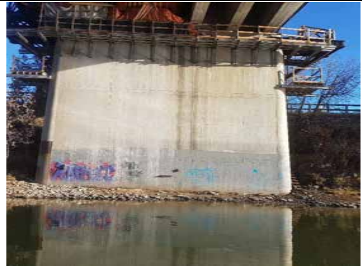
Plate 26: Looking at the north pier of the Groat Road Bridge
