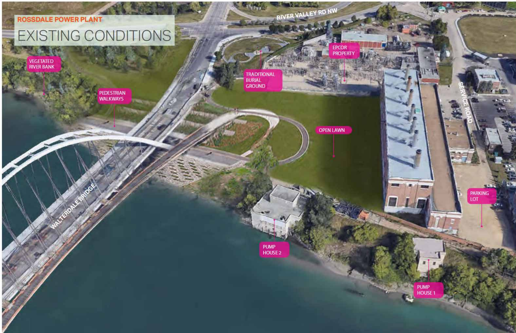
Figure 3. Rosedale Power Plant - Existing Conditions
