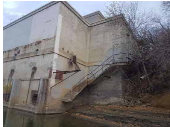
Plate 16: Looking at the downstream side of Pumphouse 2
