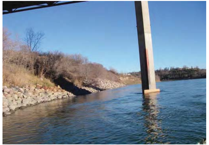
Plate 2.- Armored habitat (A2) on RUB immediately adjacent to Cloverdale footbridge (facing downstream).
