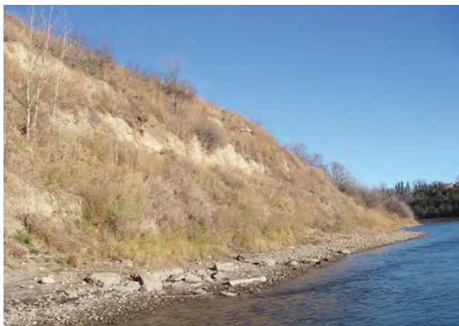
Plate 3 - Armored habitat (A1) along RUB 0.4 km downstream of Cloverdale Bridge.
