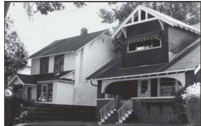
Single detached residences in Sub Area 1
