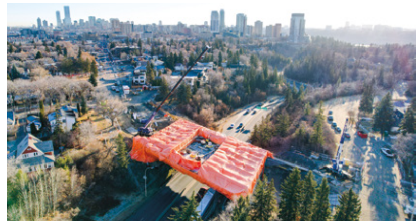
Construction on the new Stony Plain Road Bridge, November 2023
