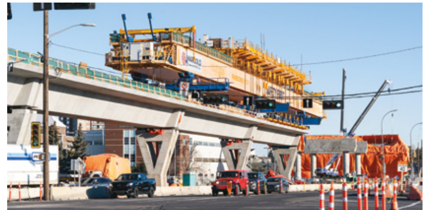
Gantry crane on the elevated guideway along 87 Avenue, November 2023
