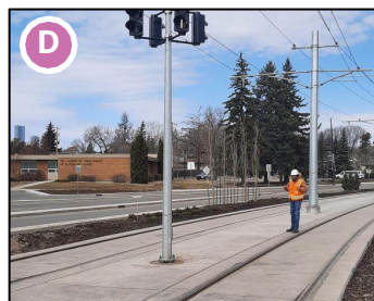
Area 3 - LRV signal testing
