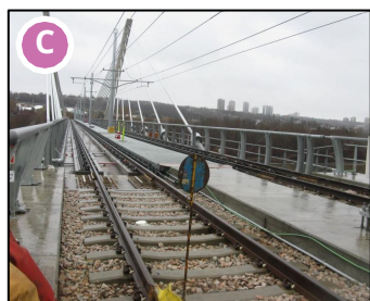
Area 2 - Rail-level view of Tawatinâ Bridge
