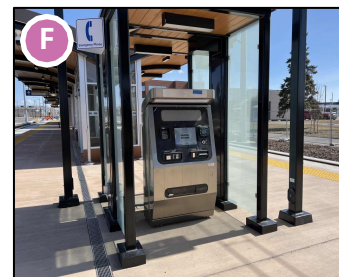
Area 6 - Ticket vending machine installation at Mill Woods Stop
