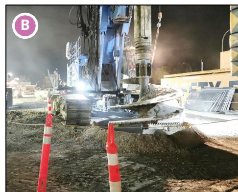
Area 6 - Drilling for piles at WEM Station
