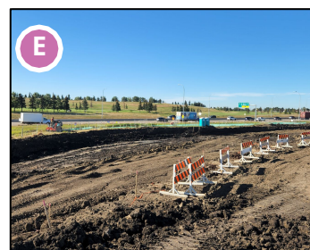
Area 9 - Earthworks continuing at OMF - Parcel B
