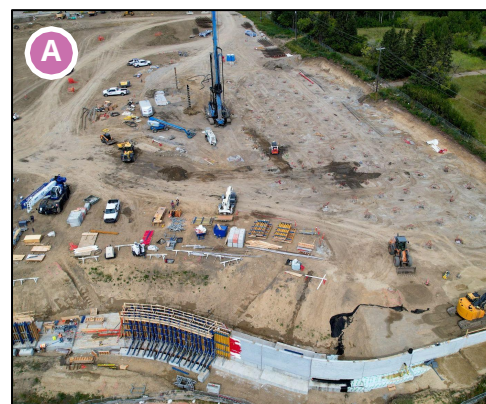
Area 8 - Retaining wall construction at Lewis Farms
