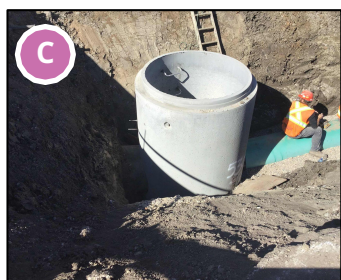
Area 5 - Drainage installation on Meadowlark Road
