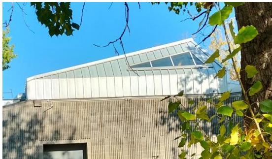
Fig. – Roof windows elephant main building
