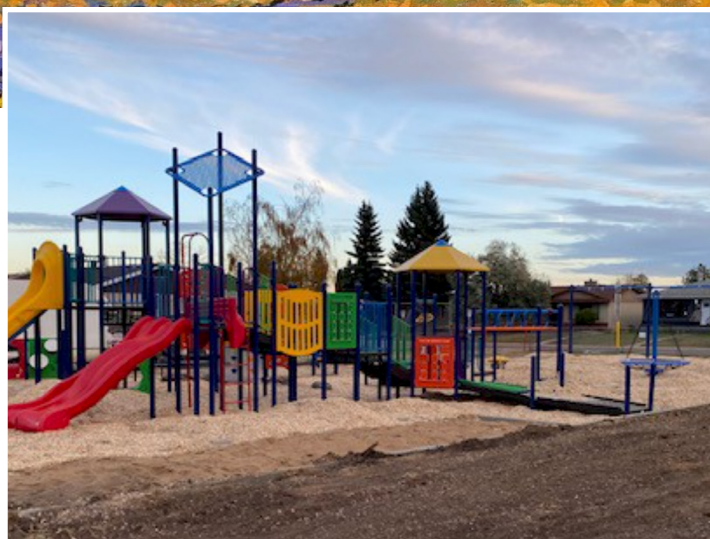
Princeton School playground redevelopment, October
