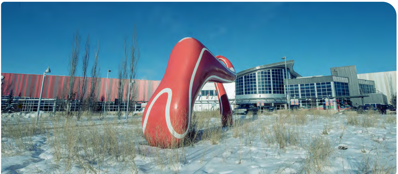
Terwillegar Community Recreation Centre
