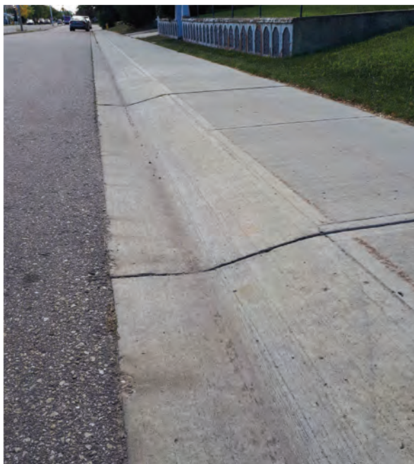
Figure 3.28 Roll Face Curb
