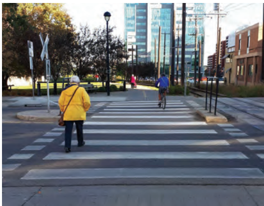
Figure 3.69: Mid-Block shared pathway Crossing
