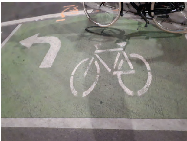
Figure 3.81 Two-Stage Turn Queue Boxes
