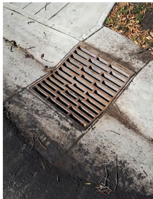
Figure 3.29 - Example of bicycle-friendly catch basin design
