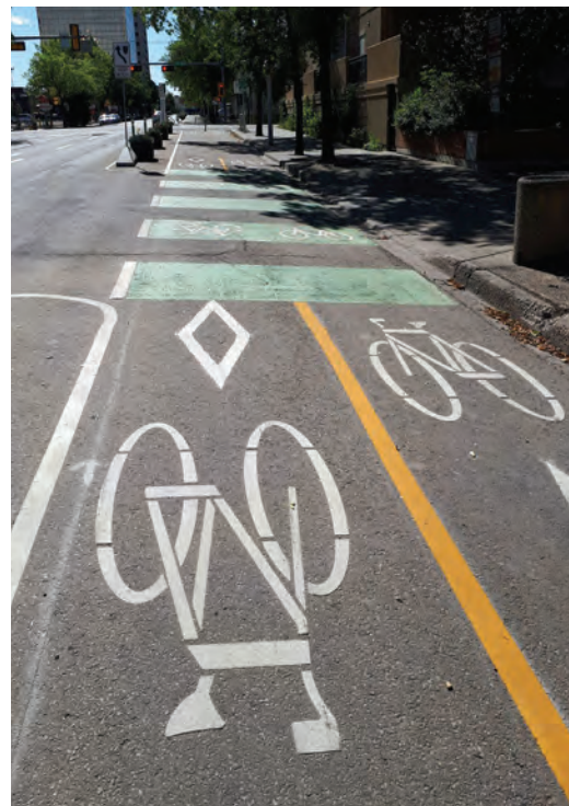
Figure 3.24 Contraflow Bicycle Lane Line
