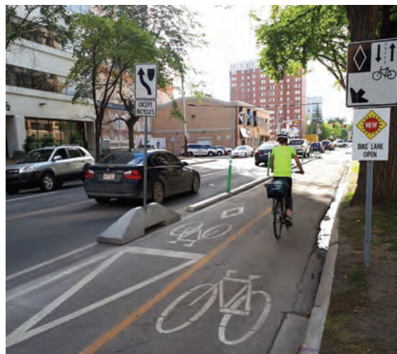
Figure 3.13 Bidirectional Protected Bike Lane
