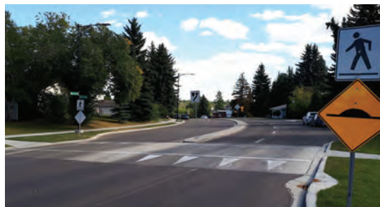
Figure 3.85 Raised Crosswalk
