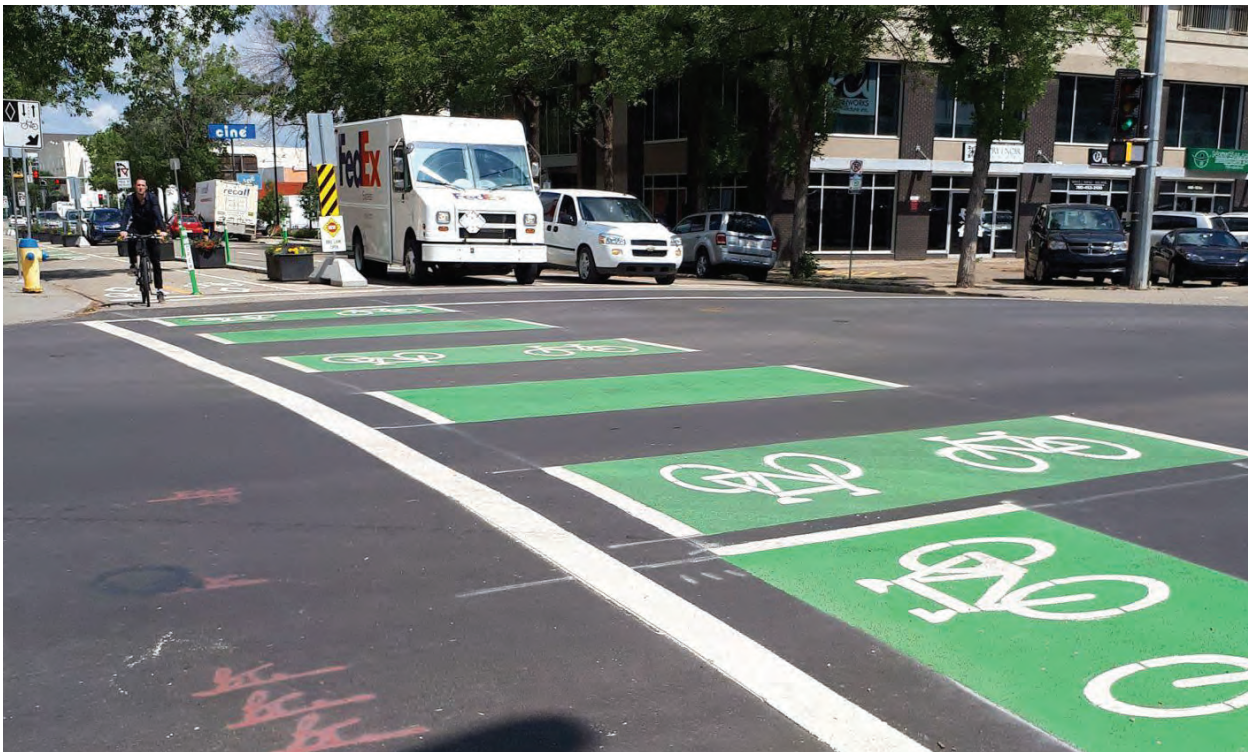
Figure 3.80 Green Coloured Conflict Marking Pavement Treatment
