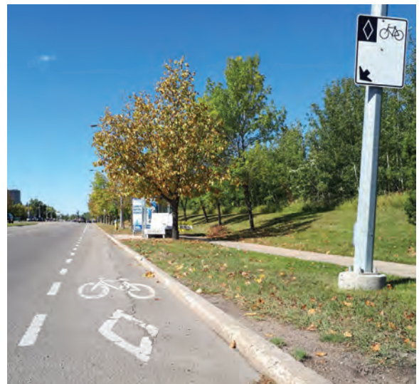
Figure 3.22 Painted Bike Lane at Curbside Transit Stop
