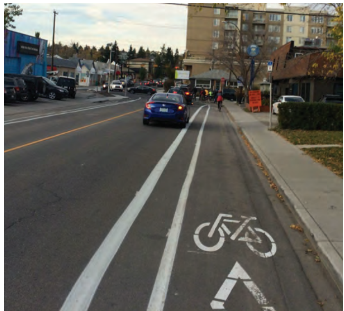
Figure 3.16 Painted Buffered Bike Lane (Source: City of Calgary)
