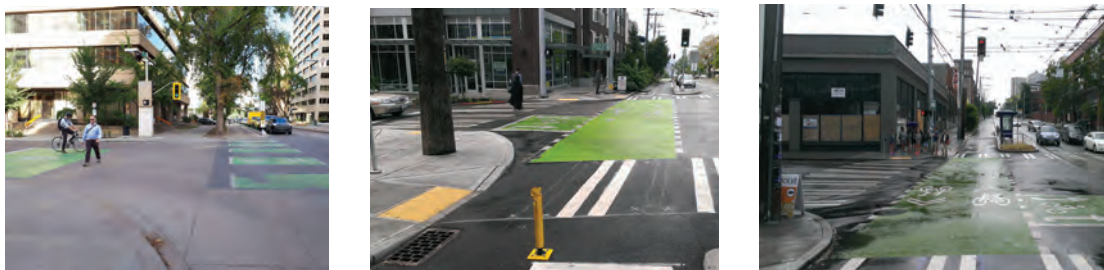
Figure 3.62 Two-Stage Left Turn Queue Boxes
