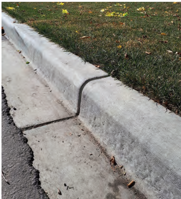
Figure 3.26 Straight Face Curb
