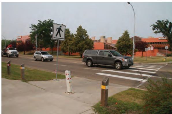
Figure 3.77: Typical Crosswalk Pavement Markings
