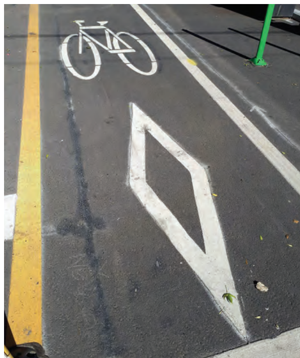
Figure 3.23 Reserved Lane Pavement Markings for Bicycle Lanes
