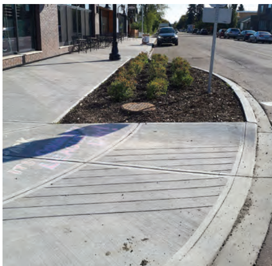
Figure 3.32 Curb Extension in Ancillary Zone
