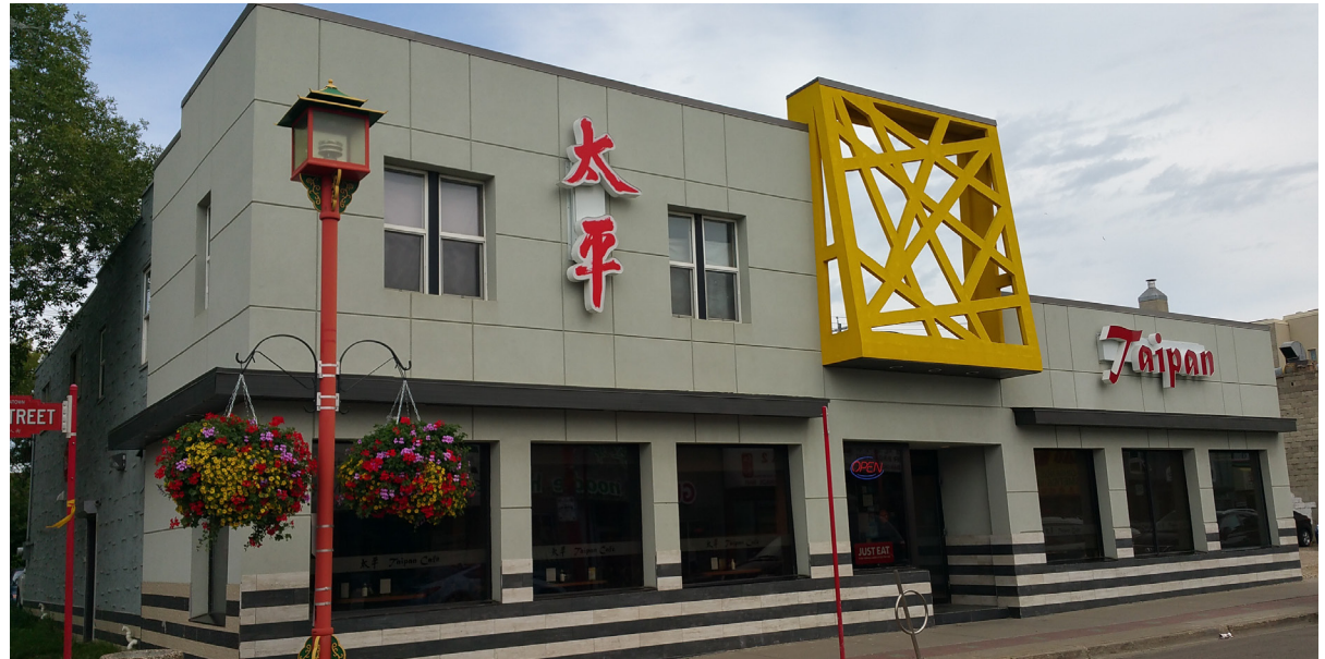
Taipan Cafe, 97 Street, Edmonton (City approved facade improvement project)
