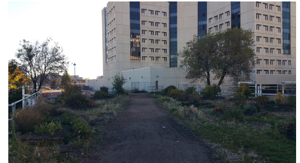
97 Street bridge (looking east)
