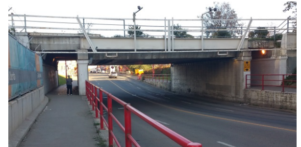
97 Street bridge (looking north)
