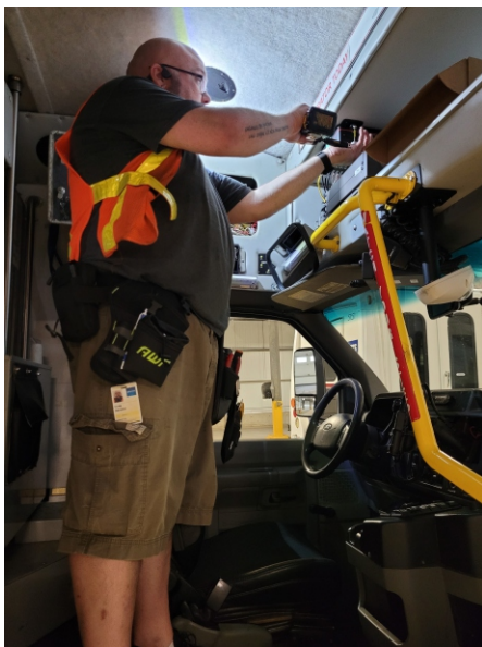
Contractor installing new router on an older bus
