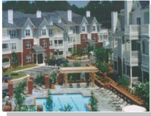
Example of an attractive multifamily development with amenities.
