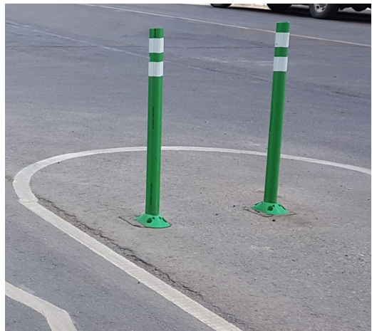
36A Avenue - Example image of flexible bollards
