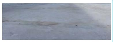
Picture of what can happen if you flood before clearing debris from rink surface. Foliage is rotting under the layers of ice and causing a swell.
