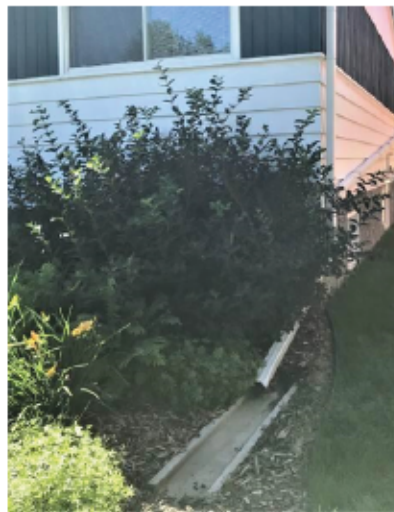
Photo 4: Roof Leader to Splash Pad Inlet
