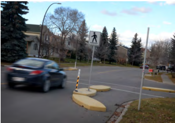
Traffic Calming Curbs 4
