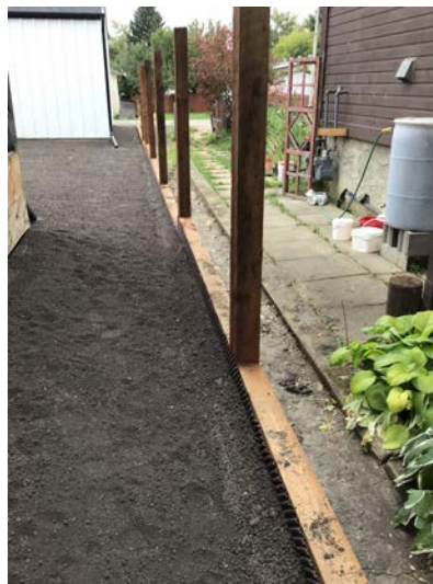
Figure 11 - Wooden retaining wall with integrated wooden fence
