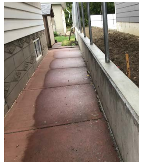
Figure 12 - Concrete retaining wall with integrated chain link fence
