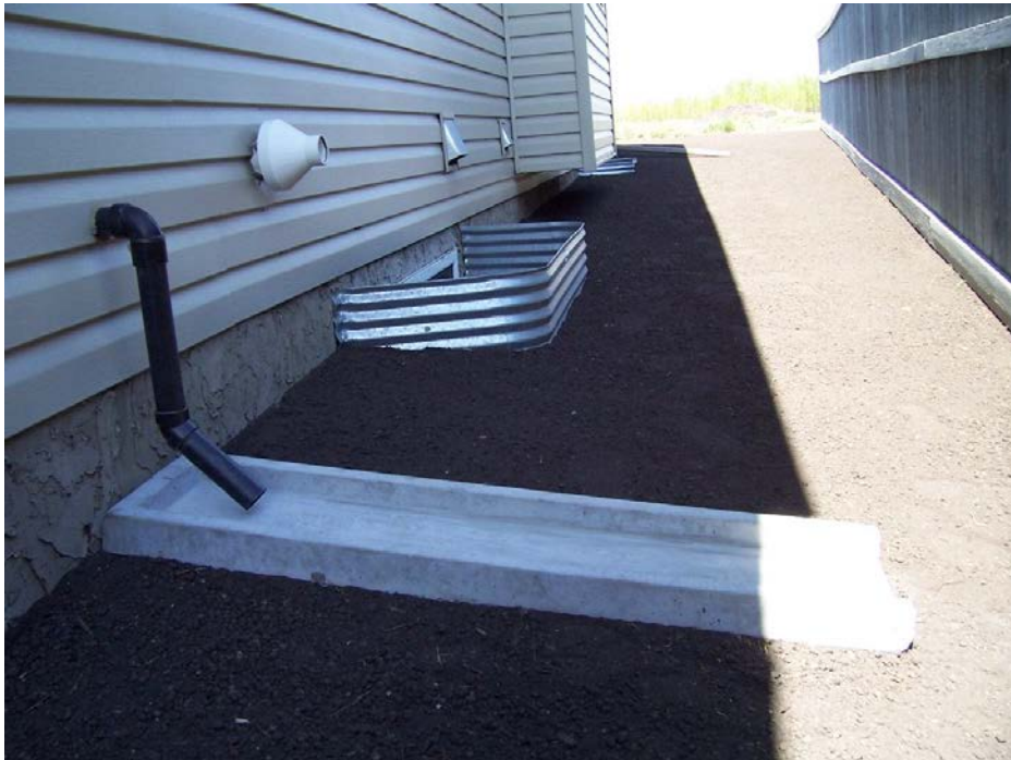
Figure 19 - Splash pad under sump discharge
