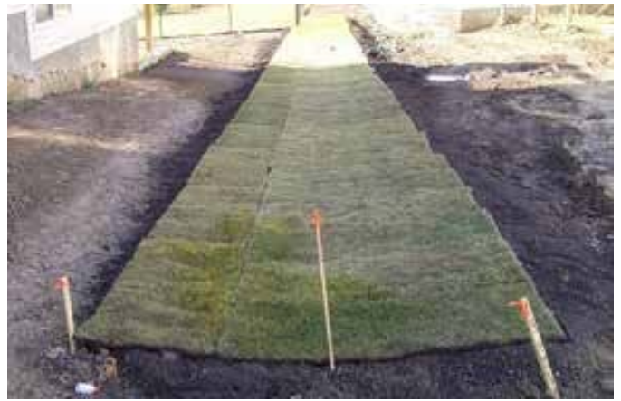
Figure 18 - Major grass drainage swale easement
