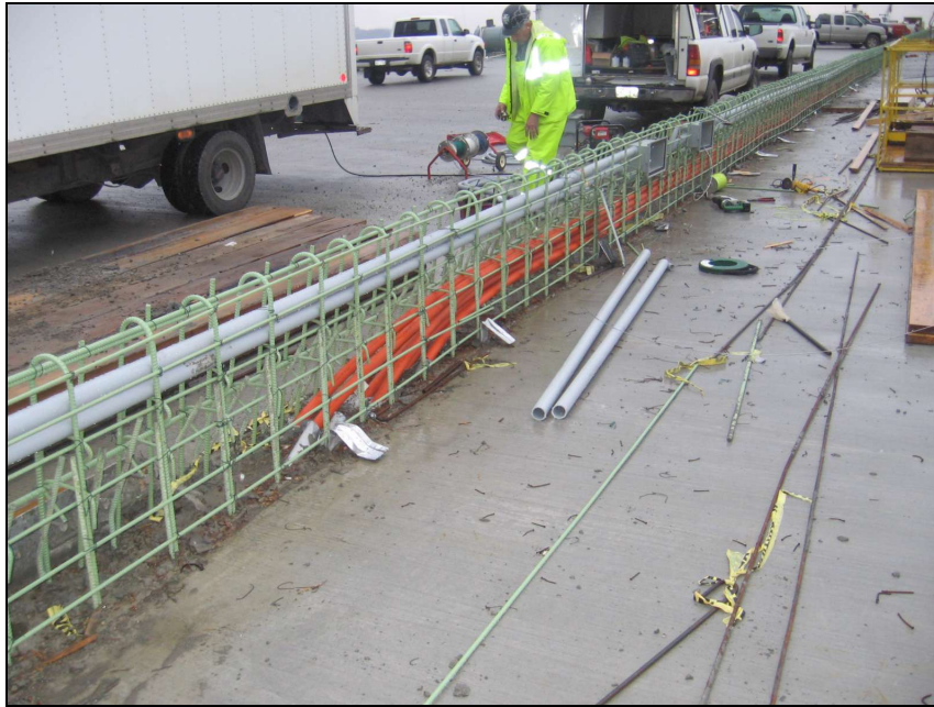
Figure 5 - Example of Conduit on Bridge Structure
