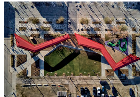
Low-impact design features include an irrigation cistern that captures stormwater run-off
