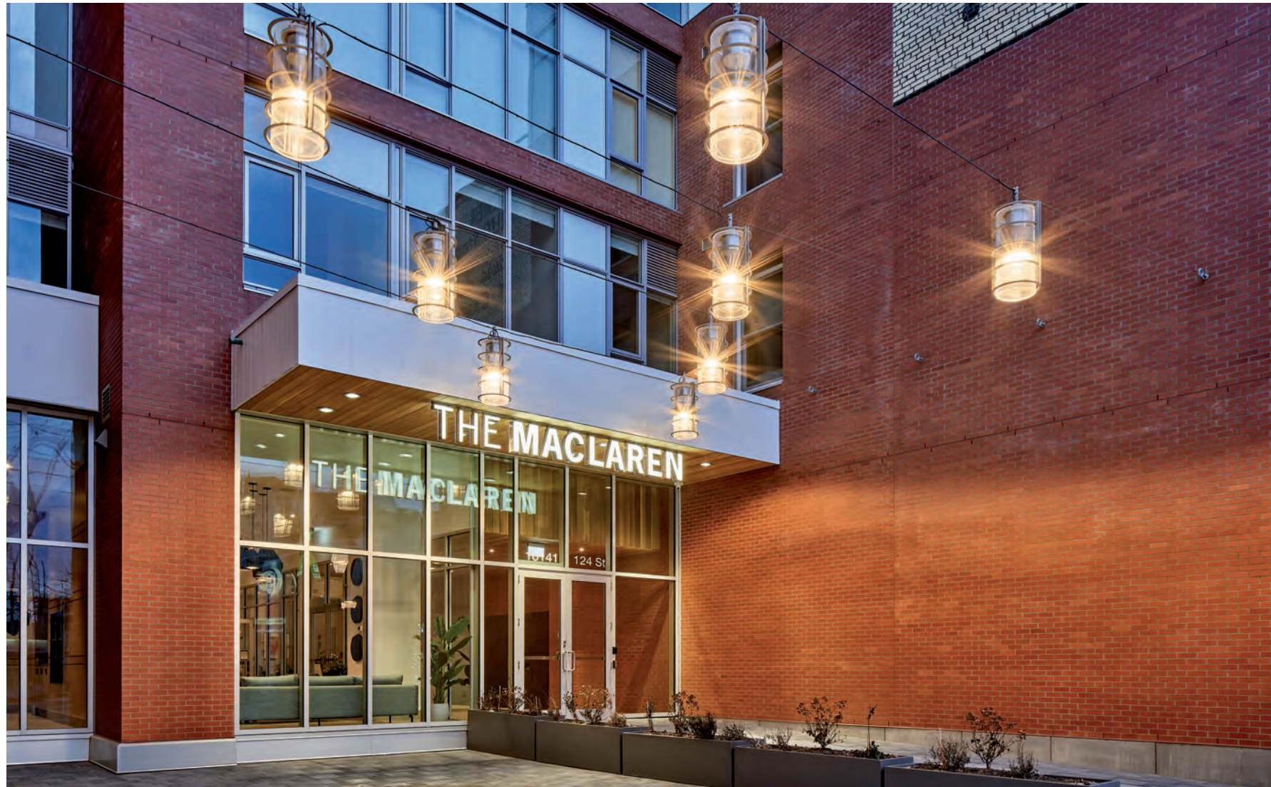
MacLaren Residential Tower entrance - modern materials inspired by historical podium next door
