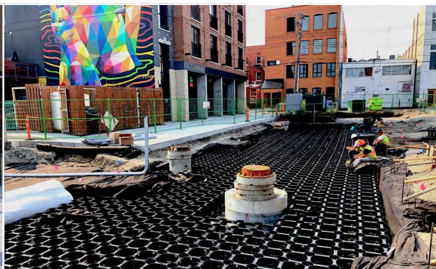
West Plaza Soil Cells Under Construction in 2021
