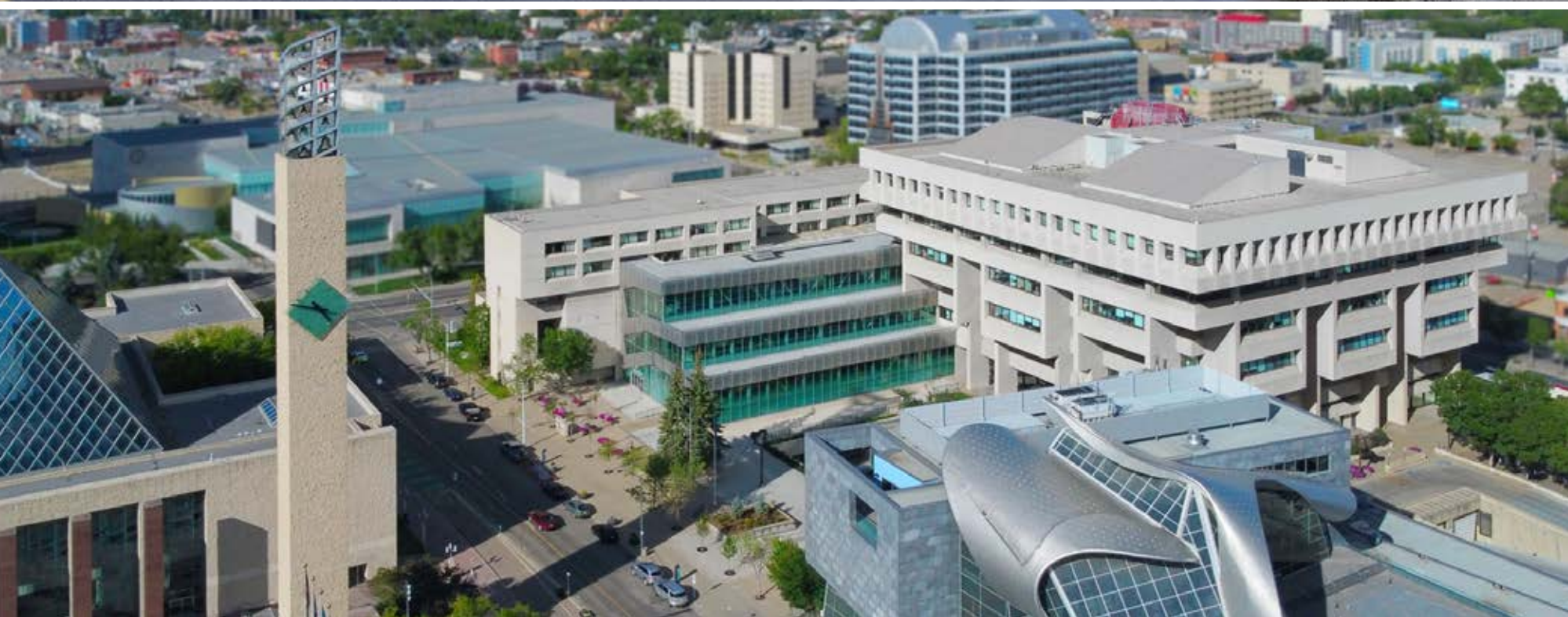
New atrium nestled between and projecting from existing law court buildings
