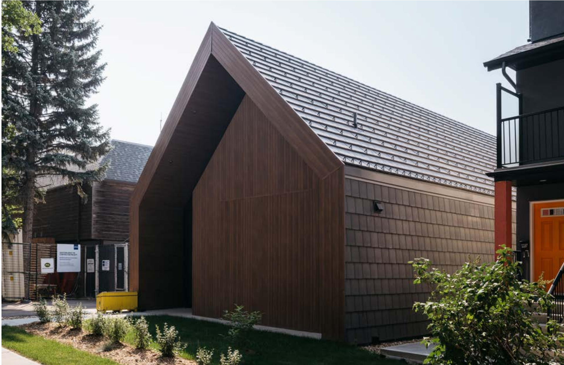
Elegant and discrete, the substation is designed not to stand out.
