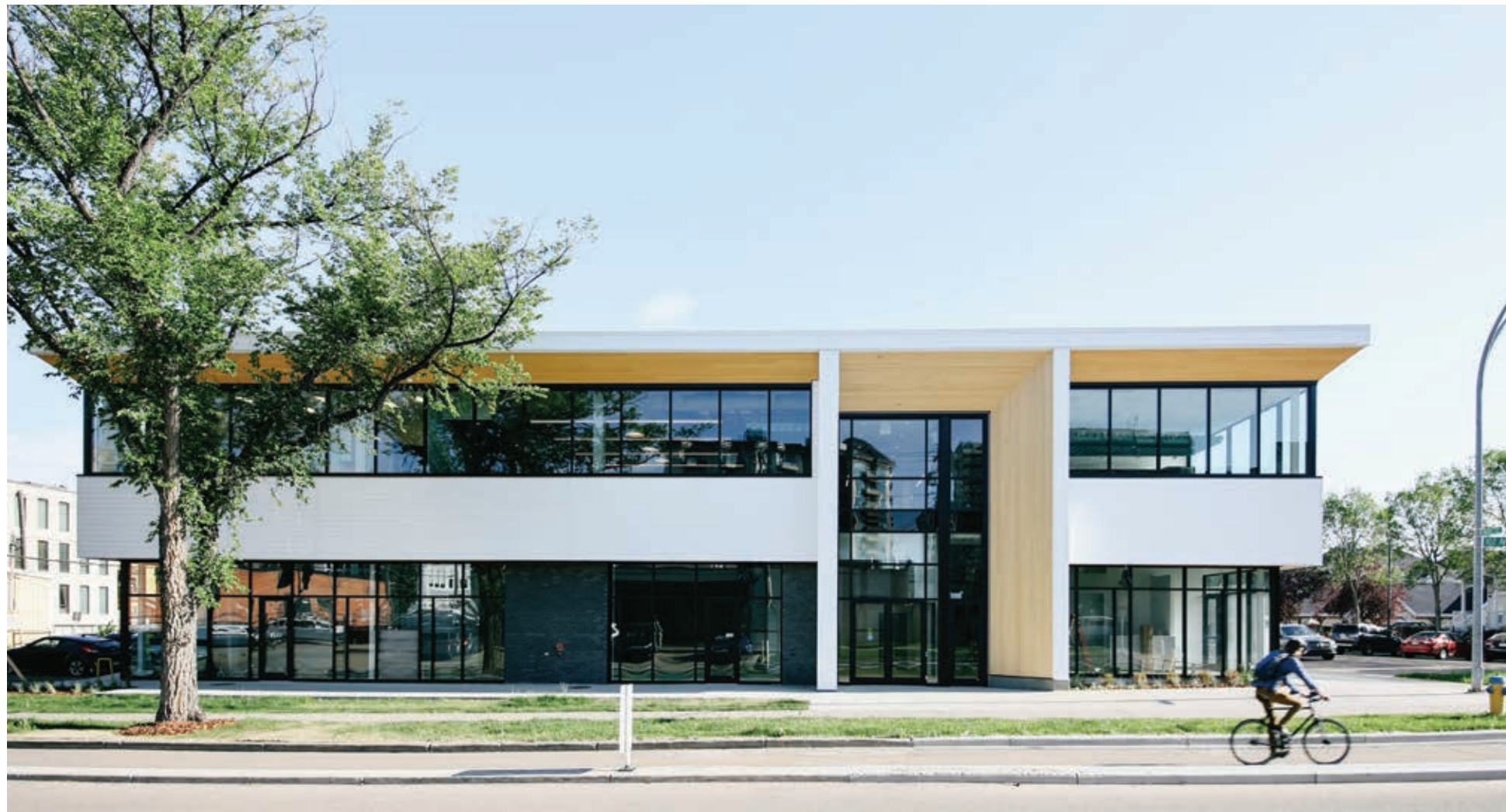
VIEW OF SOUTH ELEVATION ALONG 102 AVENUE
