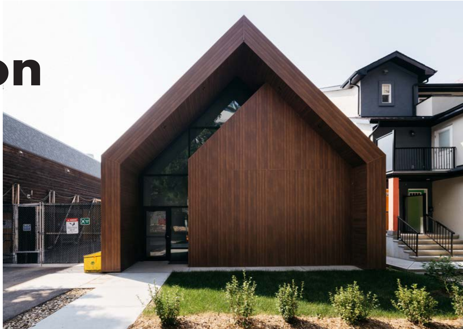
The new substation facilitates the need for new indoor electrical equipment, a switchgear.
