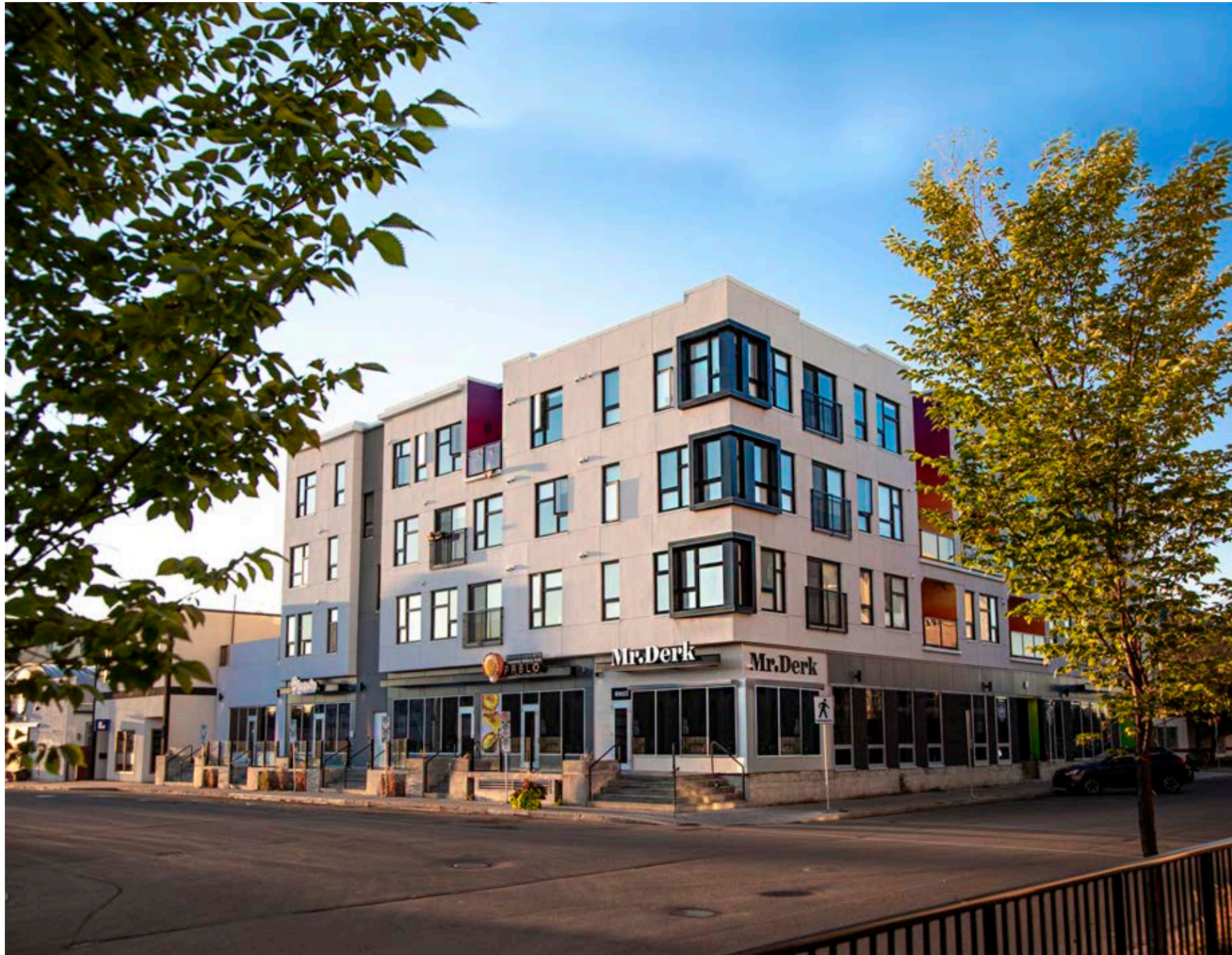
Photo - North-West View
