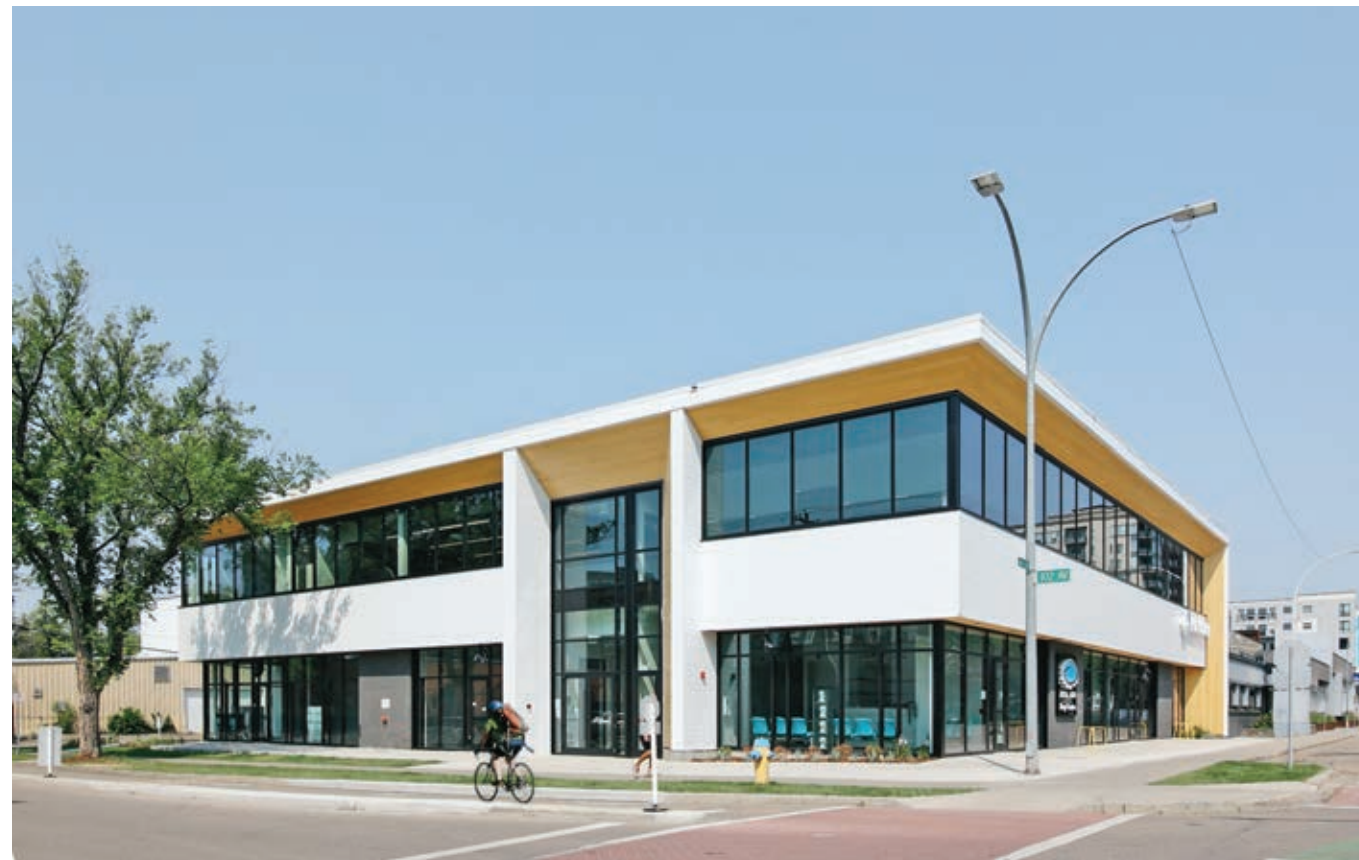
VIEW TOWARDS SOUTHEAST CORNER OF BUILDING
