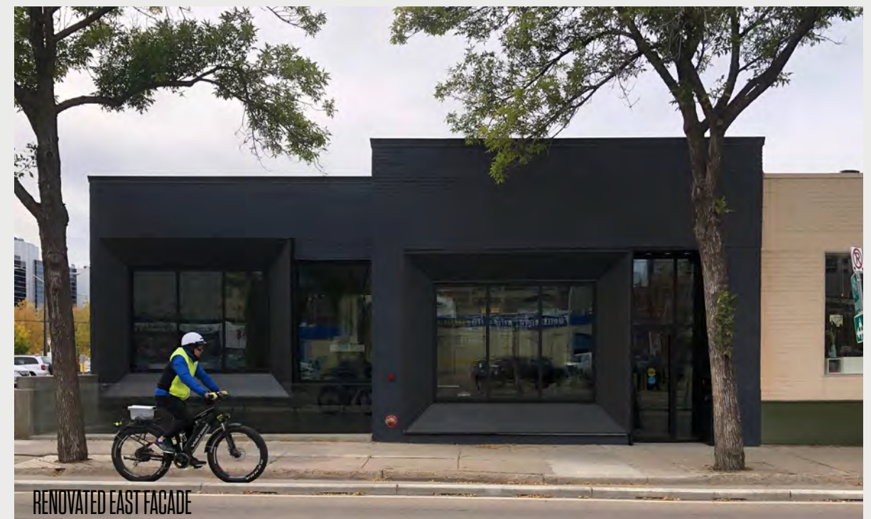
EXISTING EAST FACADE
