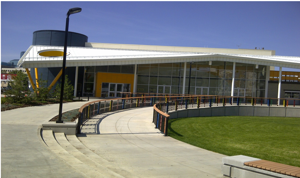
LAYING FOUNDATIONS FOR A SUSTAINABLE AND LIVEABLE CITY
