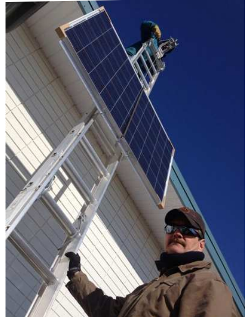
Warren Saurer, chair of the Solar Society of Alberta, helps with the installation at Meadowlark hall
