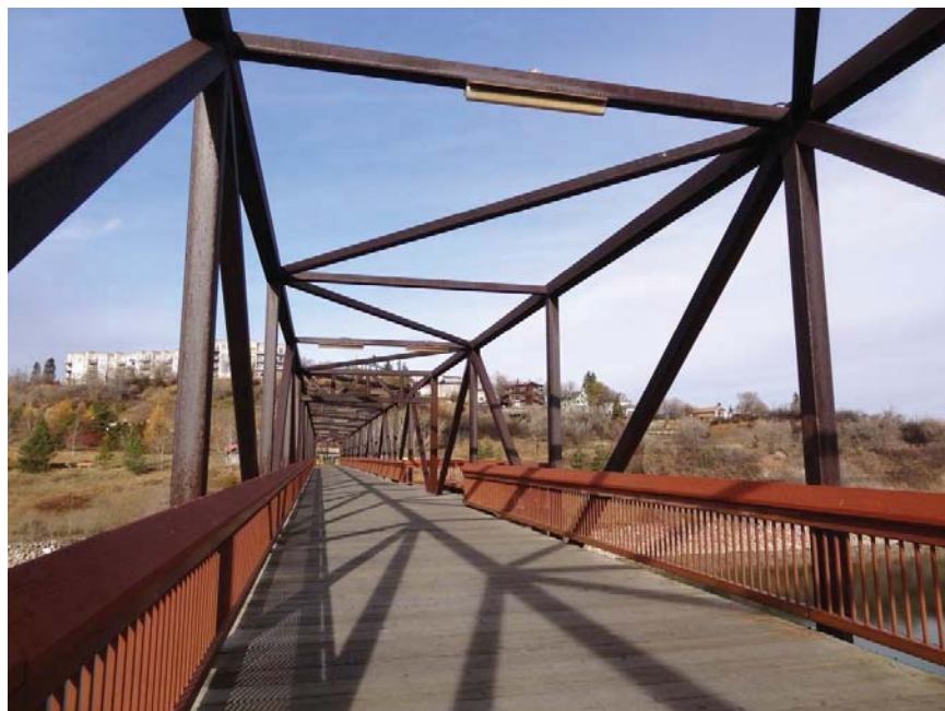
Plate 5.20. Cloverdale pedestrian bridge
