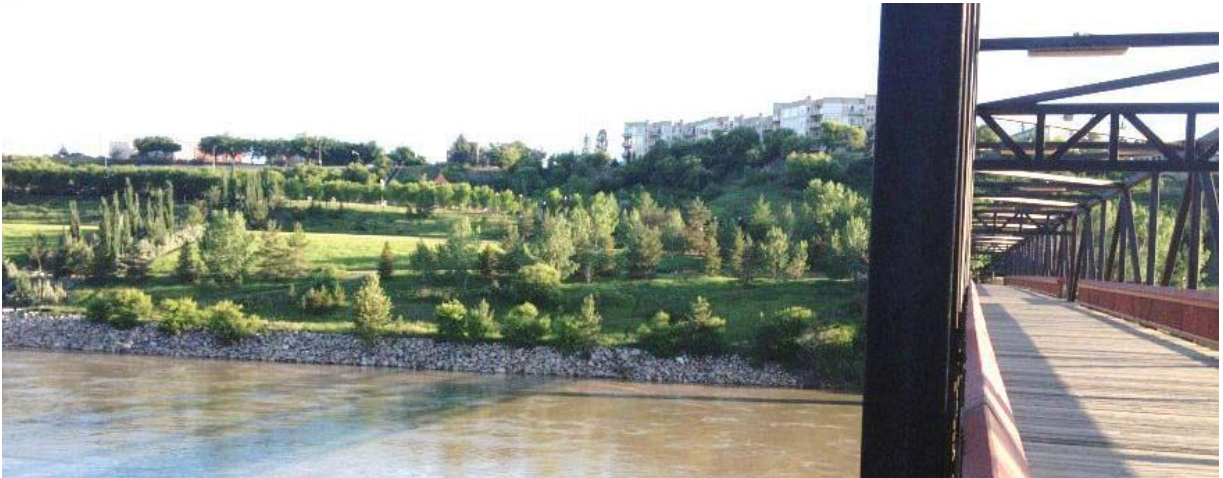
Plate 5.6. View of the armoured north bank from the Cloverdale pedestrian bridge
