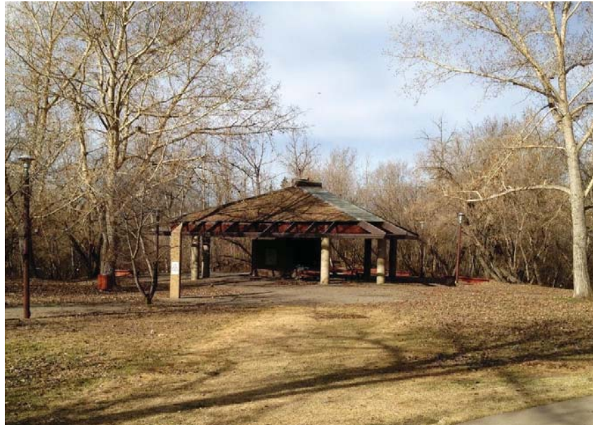
Plate 5.21. Picnic shelter at HME Park
