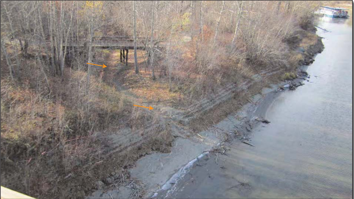
Figure 21. View facing southwest from footbridge showing gully (→) incised into thick floodplain deposits on the right bank (south side bank) of the river.
