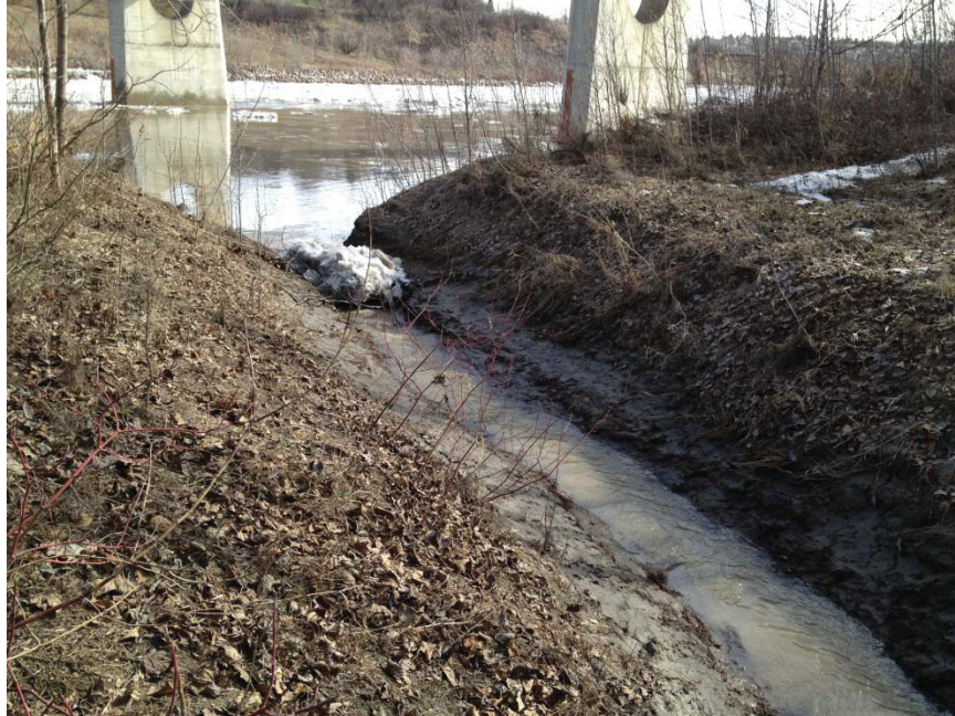
Plate 5.8. Abandoned reach of Mill Creek continues to convey water to the NSR, April 2013
