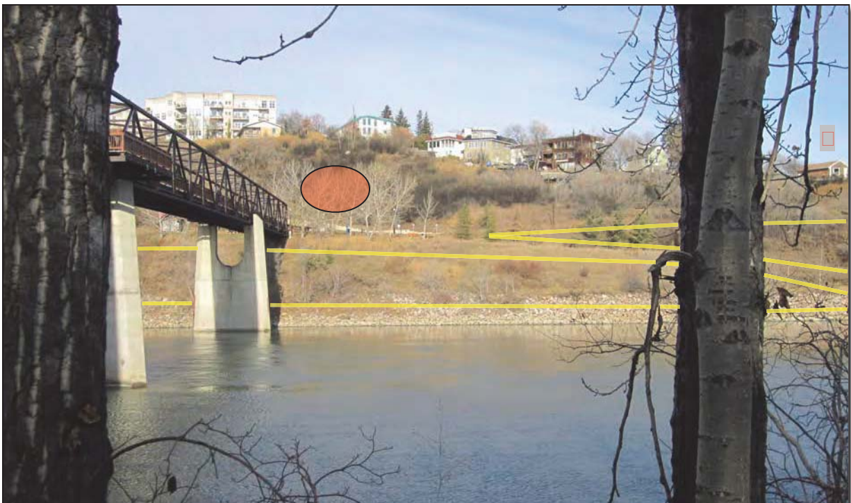
Figure 12. View facing north from south bank of North Saskatchewan River showing existing footbridge and approximate location of proposed LRT tunnel portal (●) on north valley slope. Note: bedrock likely near surface below thin vegetative/colluvial or landscaped cover (areas bounded by — lines). 1 = reference point (see house in Fig. 13)
