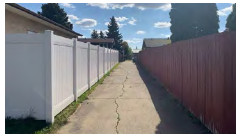
Existing utility lot
