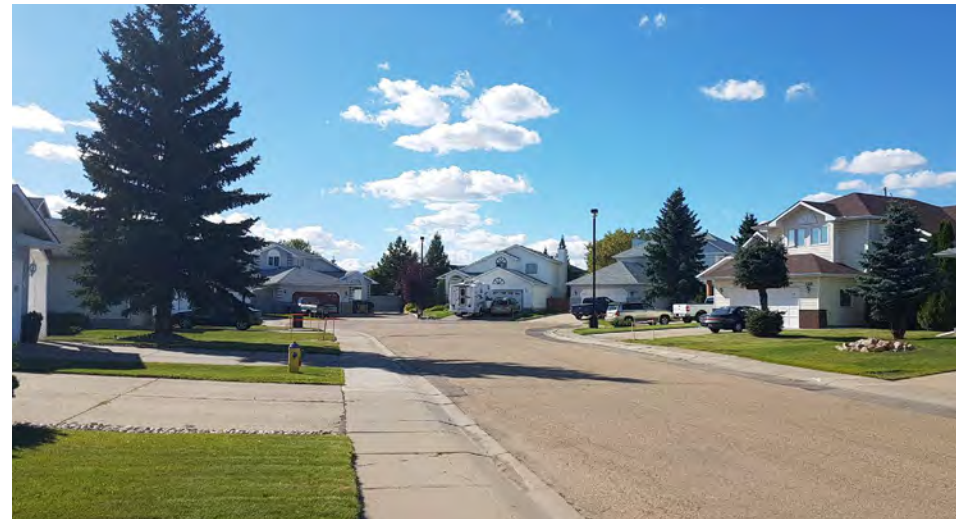
Typical Baturyn local residential road with curbside sidewalks and rolled face curbs
