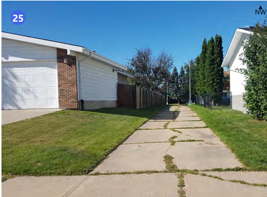
View from 168A Avenue to 169 Avenue
