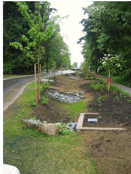
Naturalized drainage way with check dams.
