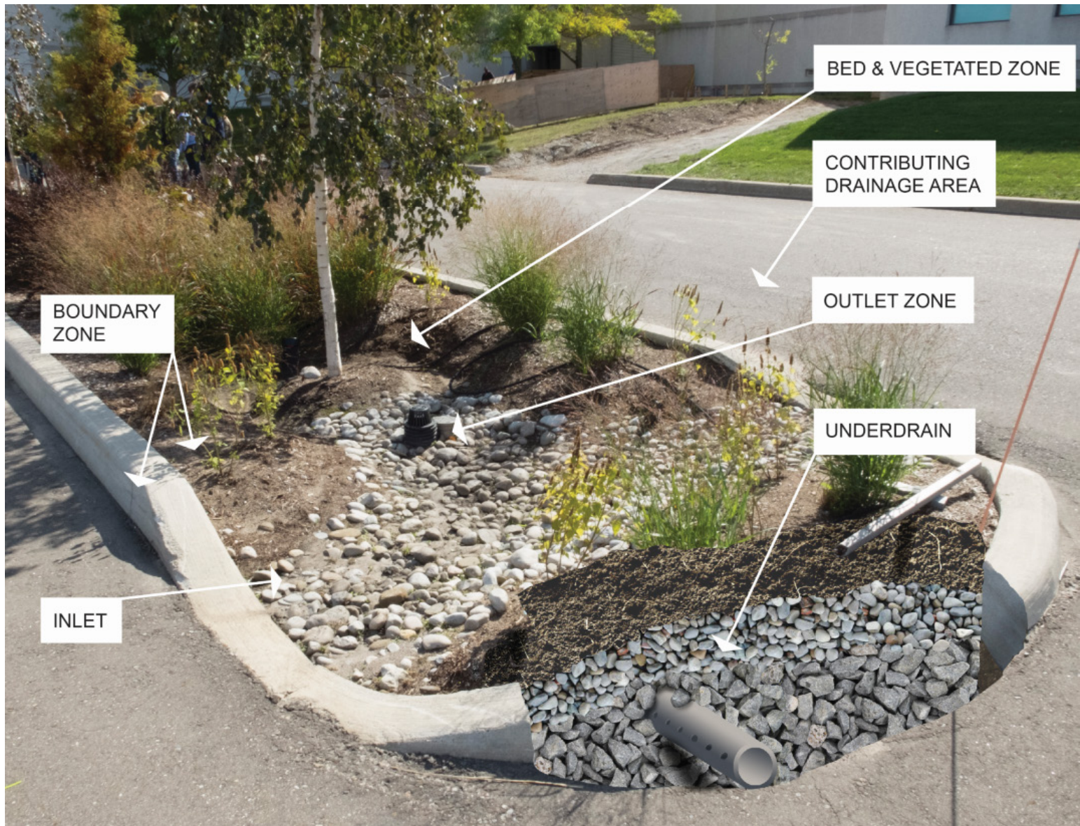
Figure 5. Bioswale Inspection Zones
