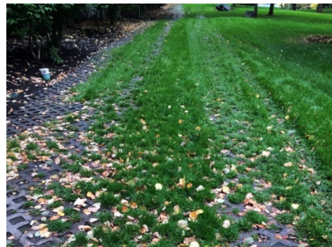
Grass pavers – dry conditions
