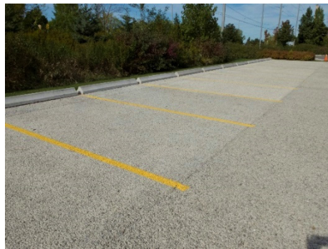
Porous concrete – dry conditions
