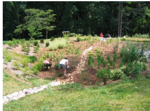
Stabilized drainage area.
