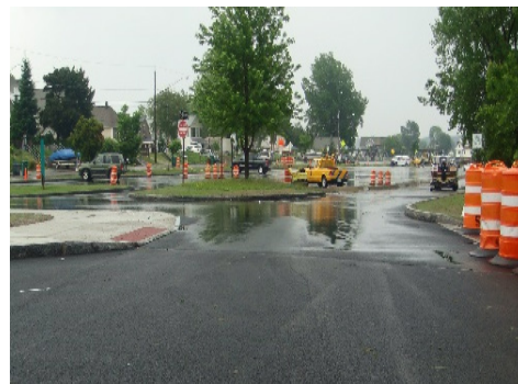
Permeable asphalt in foreground, traditional in background – wet conditions
