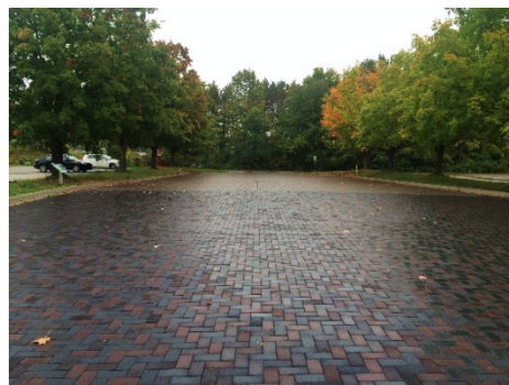
Interlocking pavers – wet conditions
