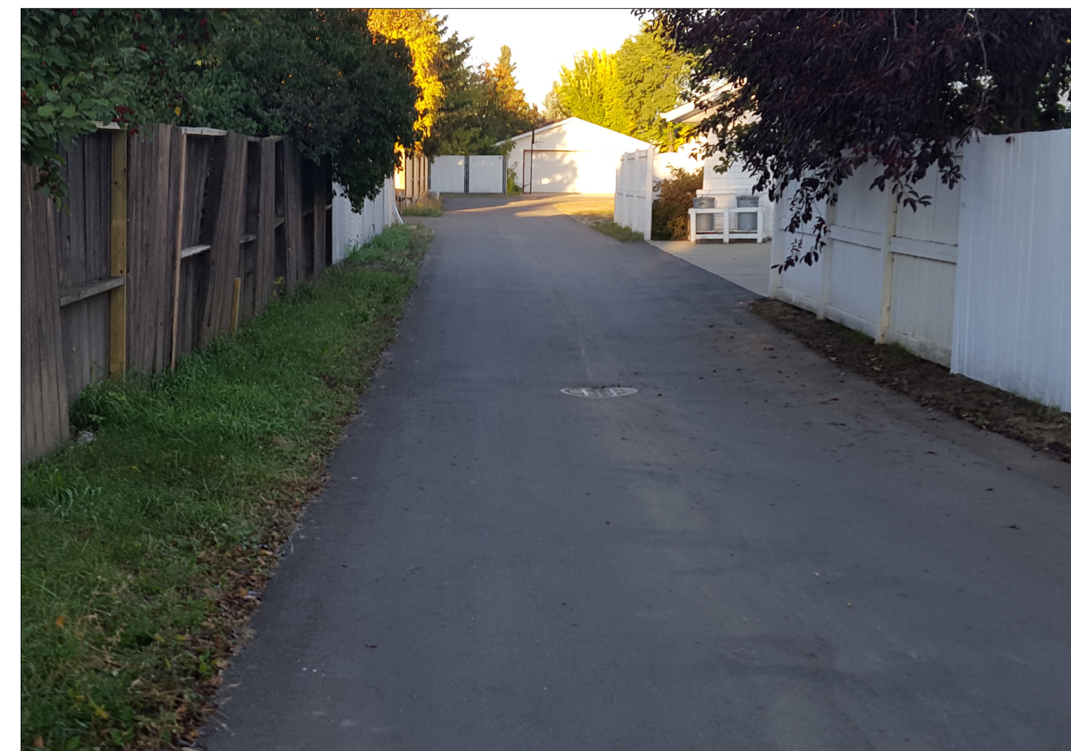
After alley renewal
