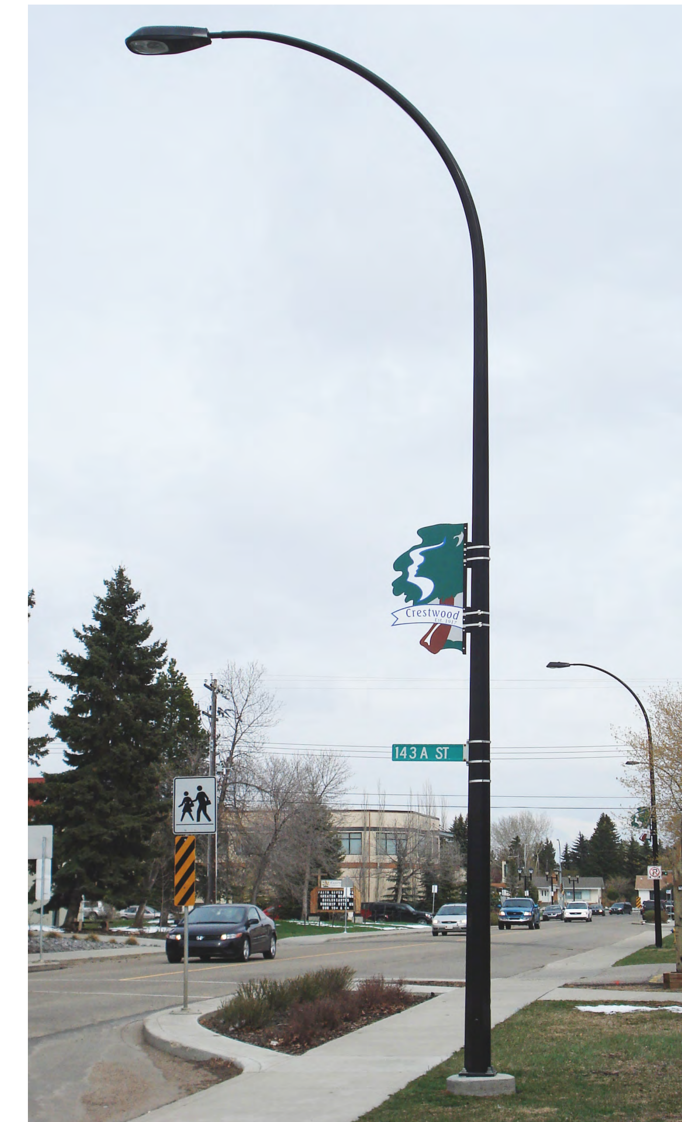
Example of Decorative street light
