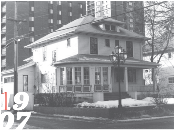
Victoria Avenue Residences- The Weinlos/Friedman Residence, 1993. (ACD)
