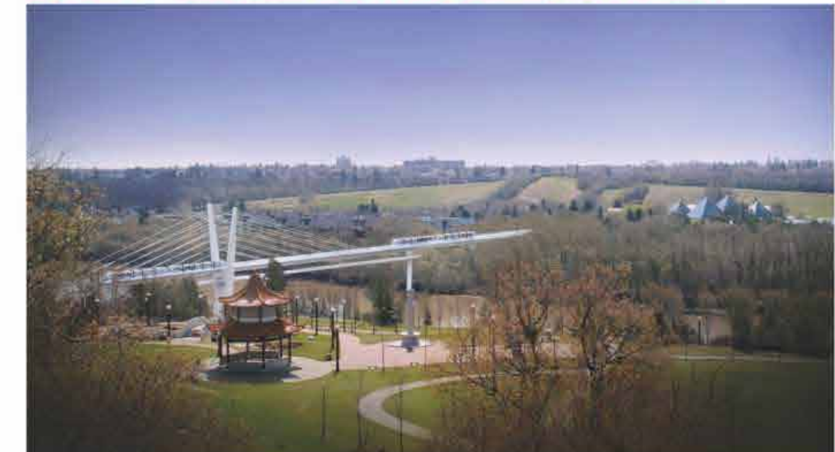
Option 2 - Extradosed bridge looking Southeast
