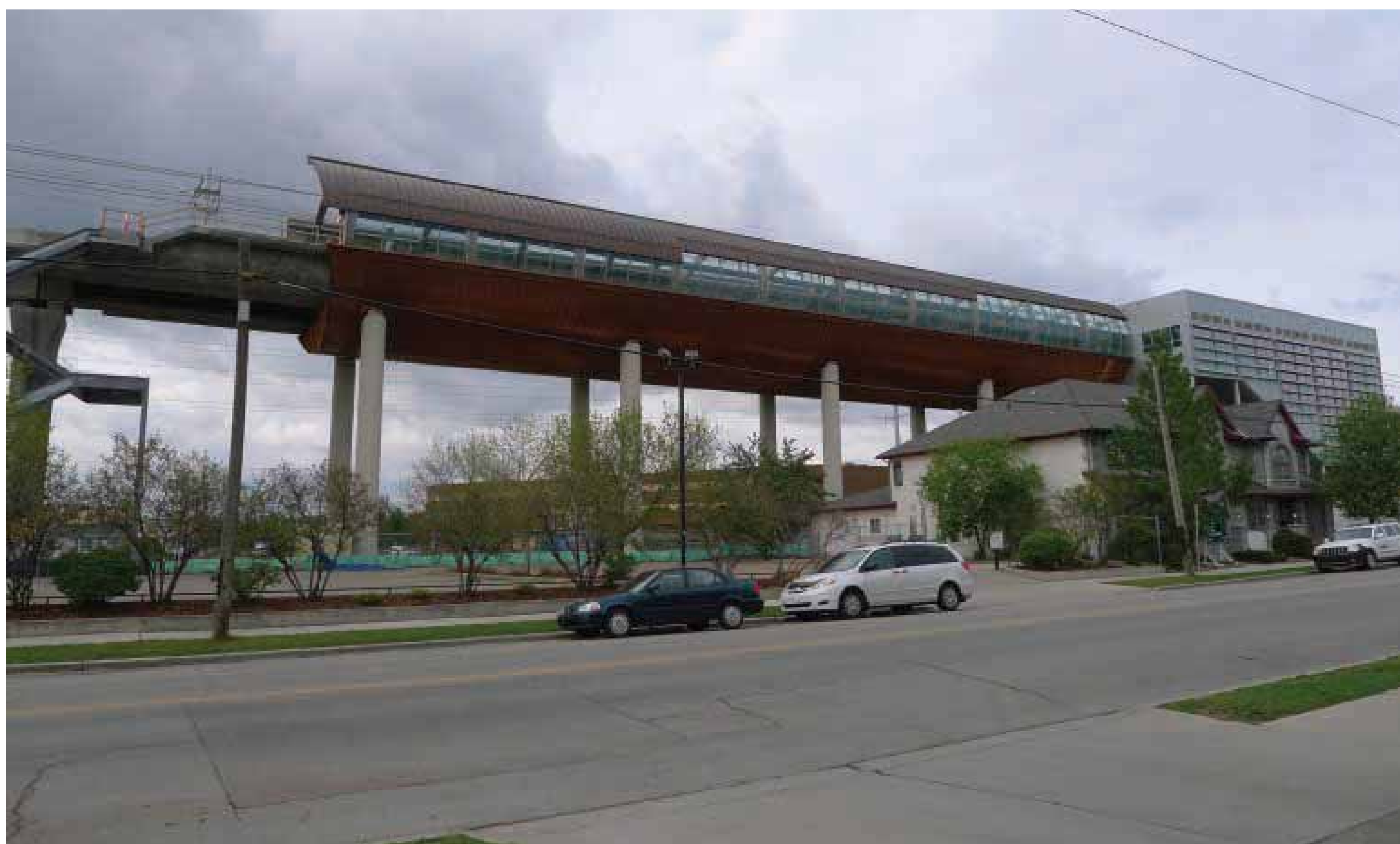
Example of an elevated station: Sunalta station, Calgary, AB
