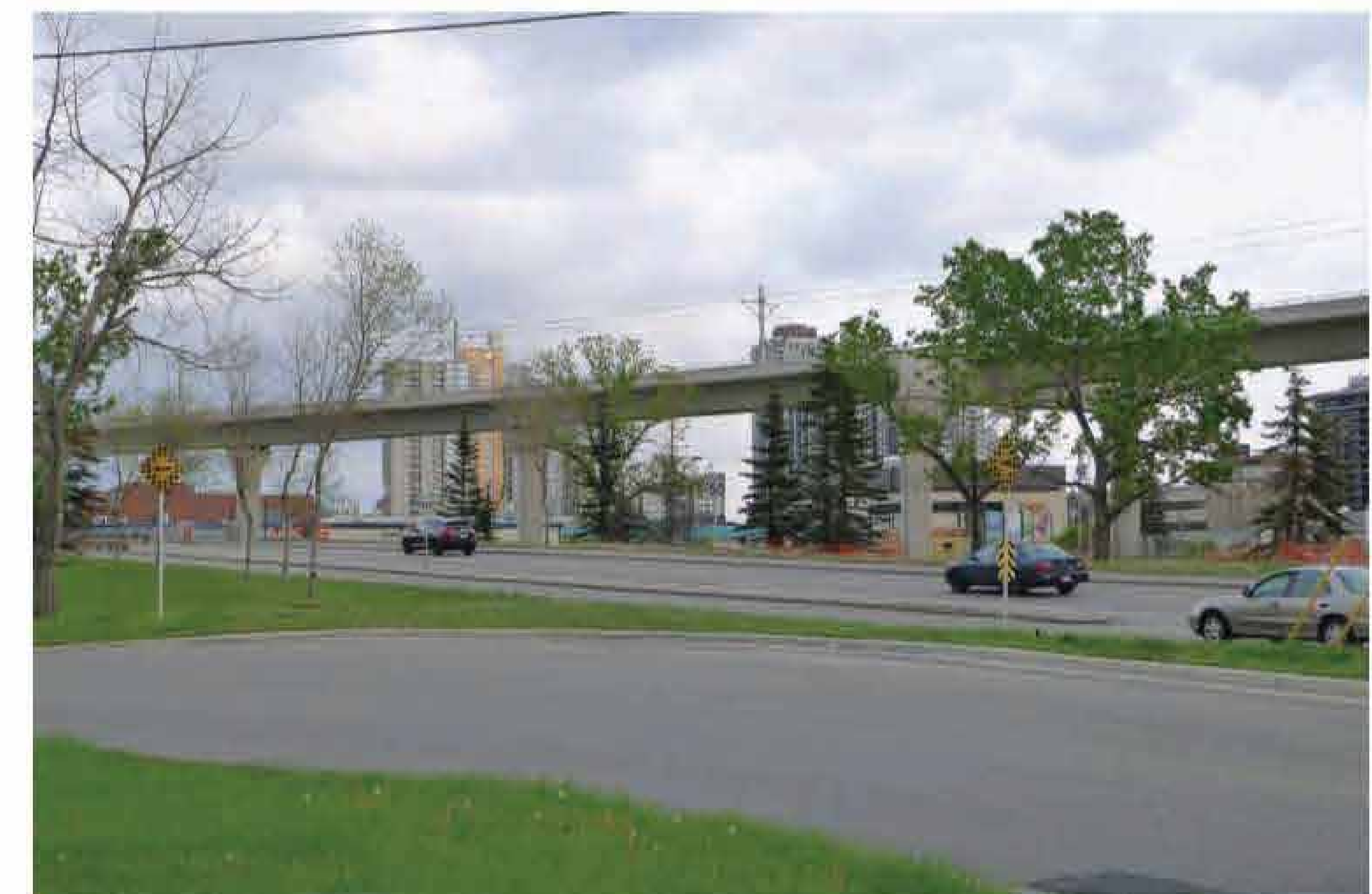
Example of elevated LRT bridge - Calgary, AB
