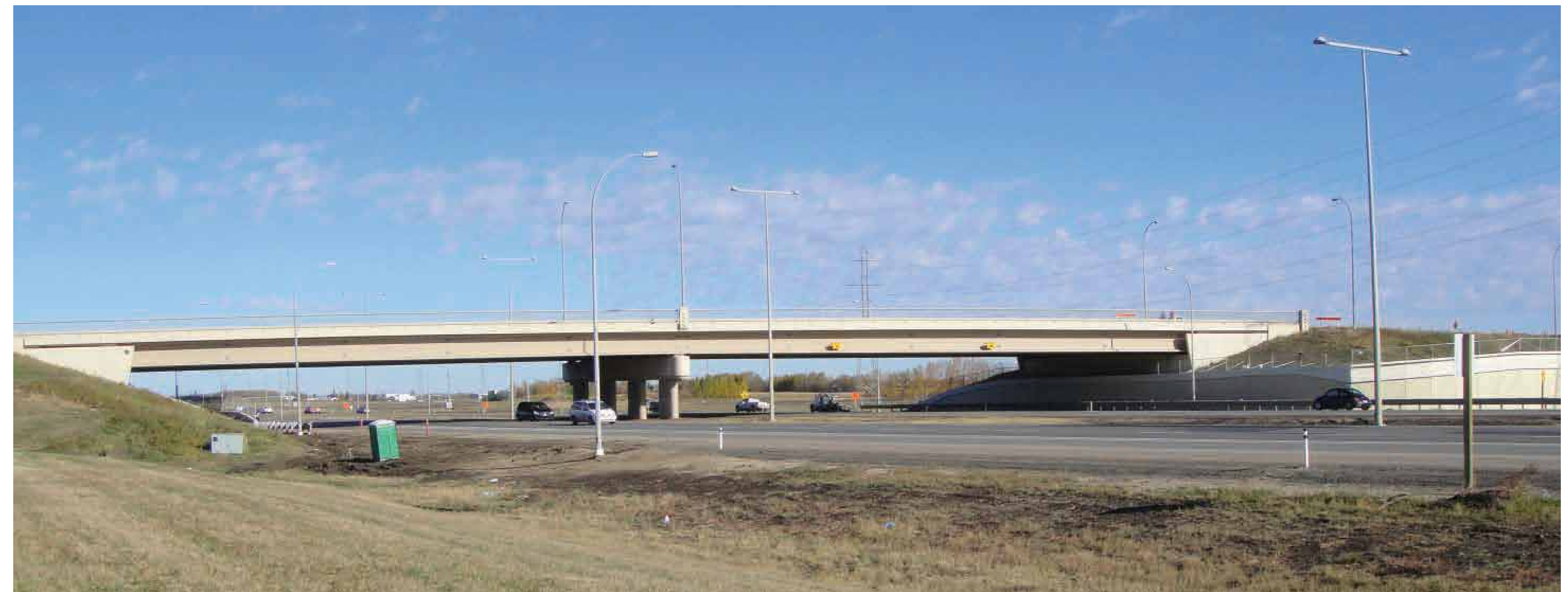
Existing 87 Avenue bridge over Anthony Henday Drive
