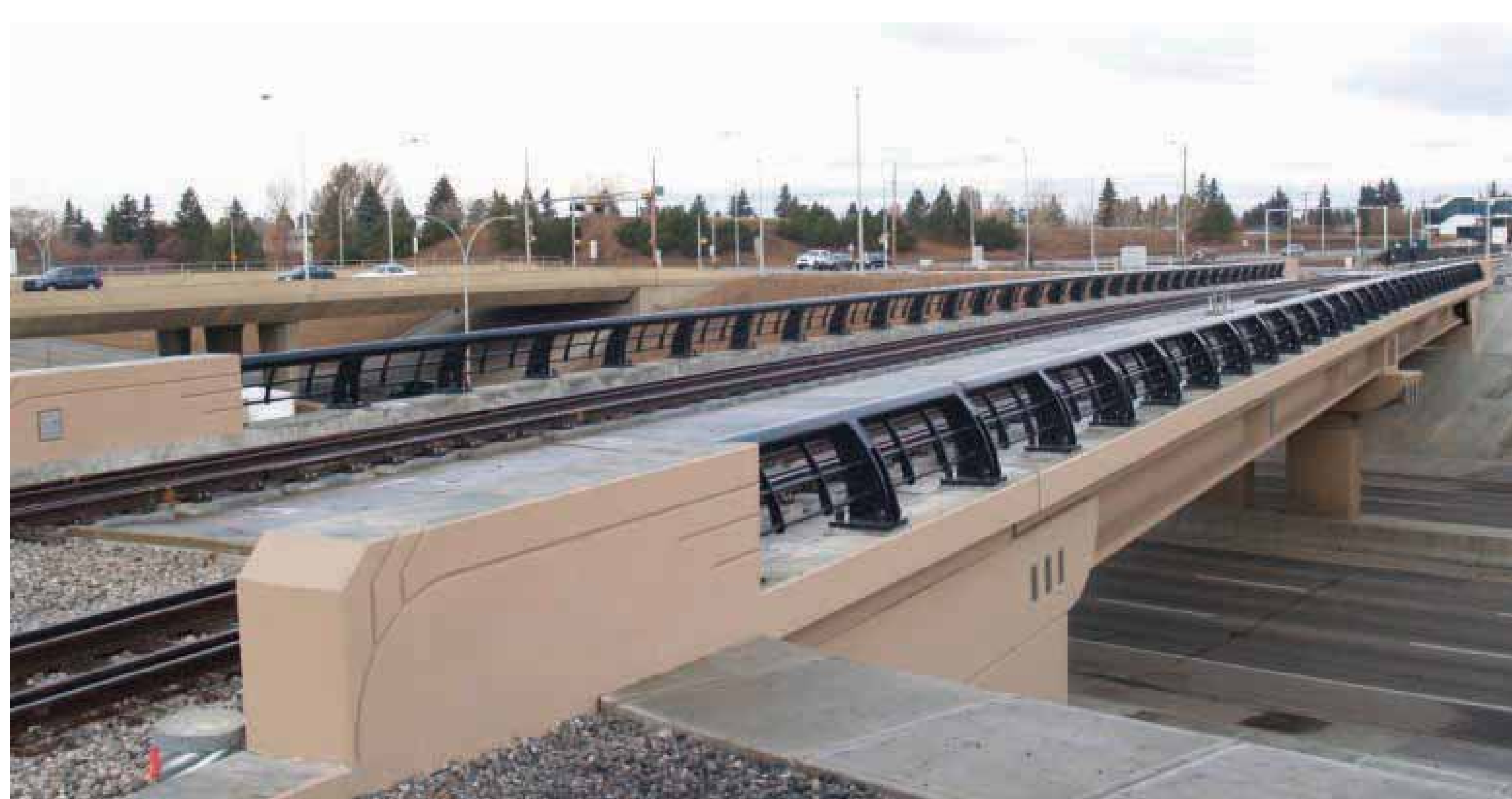
Example of Existing LRT bridge over Whitemud Drive
