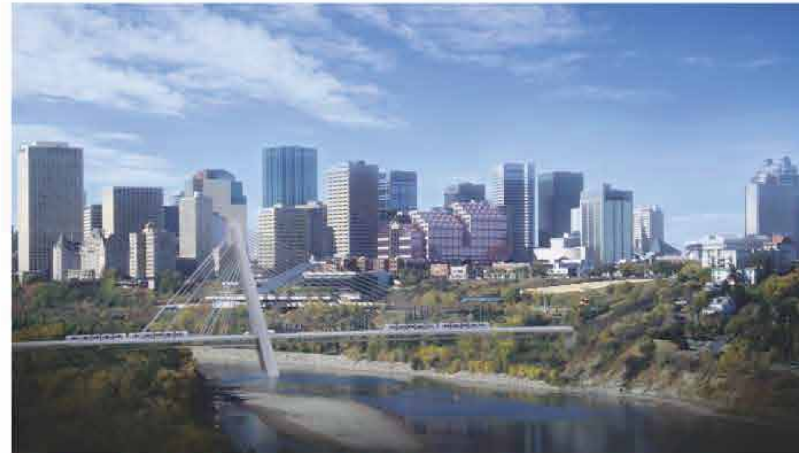
Option 1 - Cable stayed bridge looking Northwest
