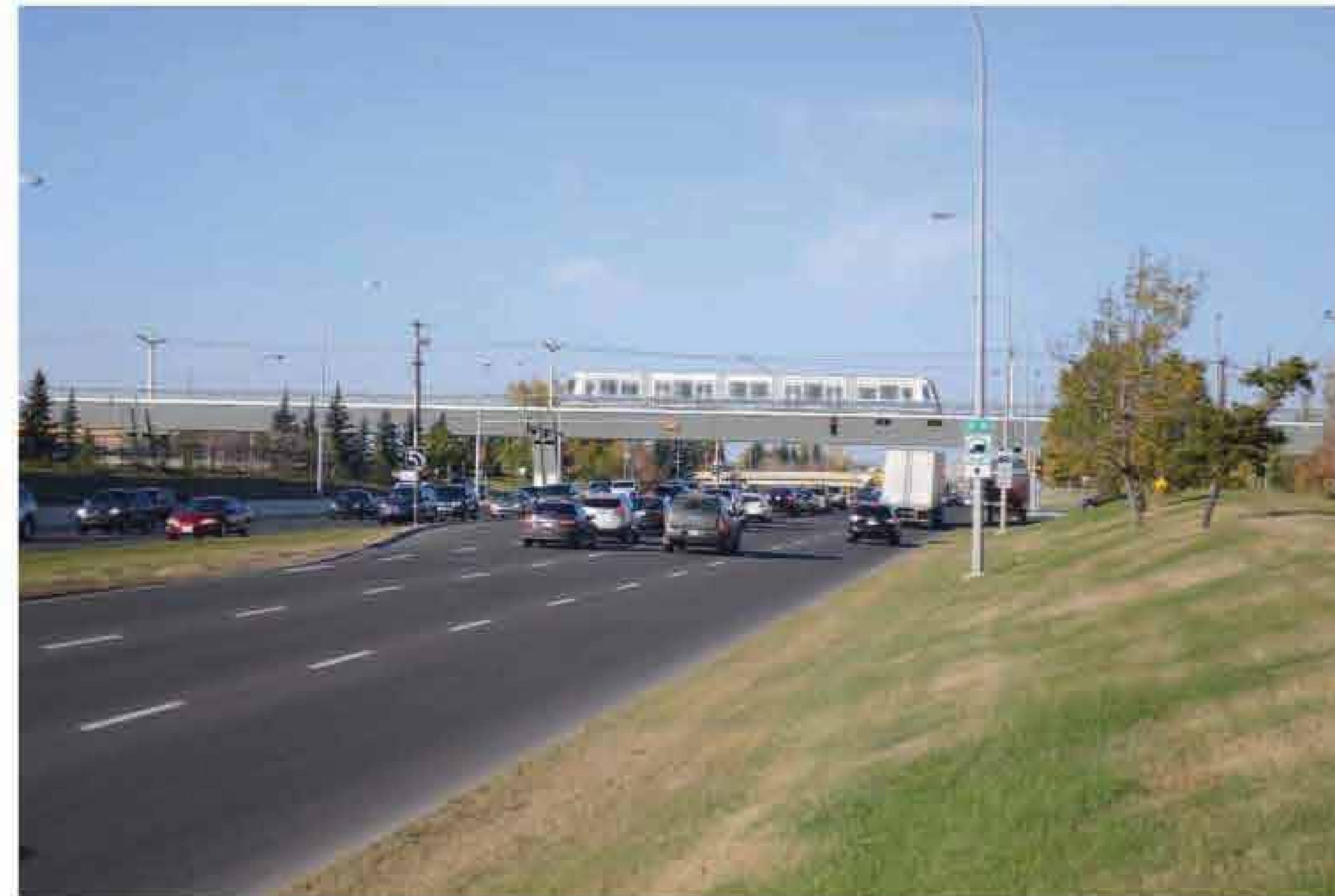
View 1 - Bridge at 170th Street/87 Avenue Intersection
