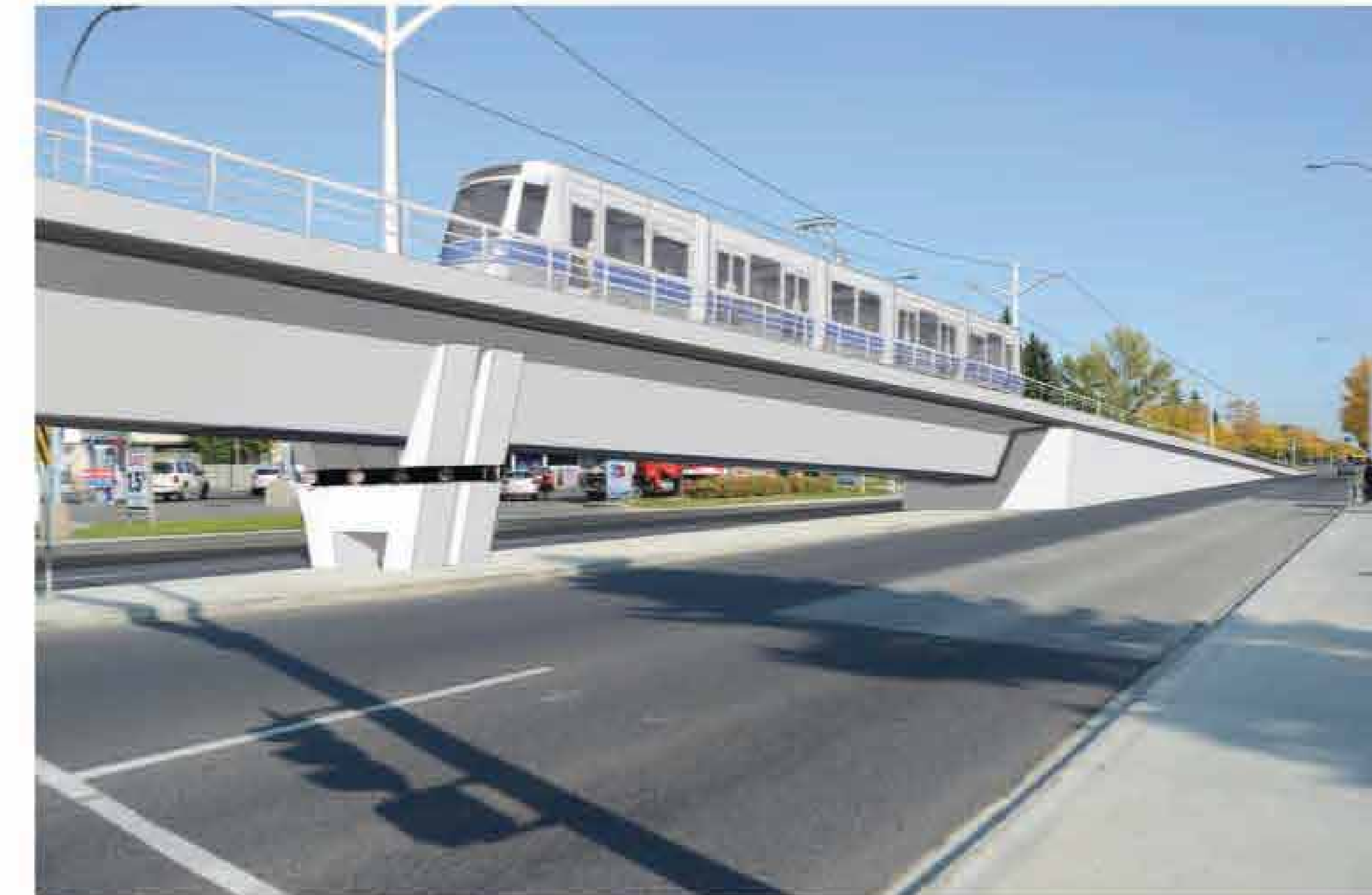
View 2 - Ramp on 87th Avenue East of 165 Street
