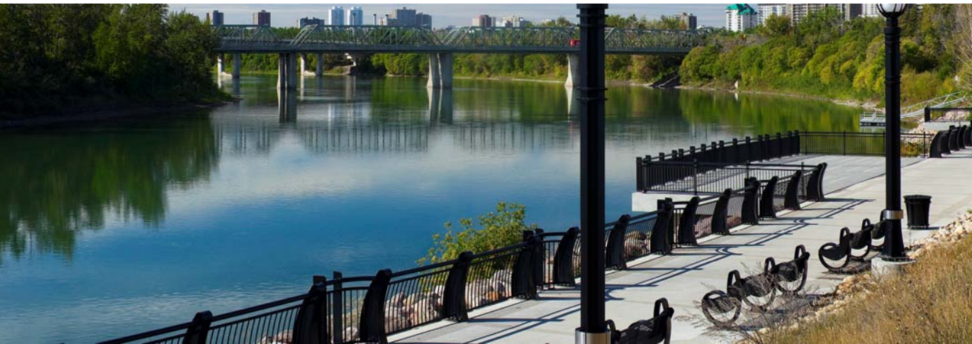
Image courtesy Carlyle + Associates
