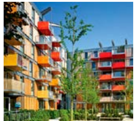
Figure 20 Medium Rise Apartments
