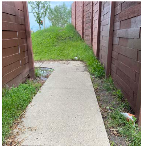
Breezeway connecting to 170 Street, looking north
