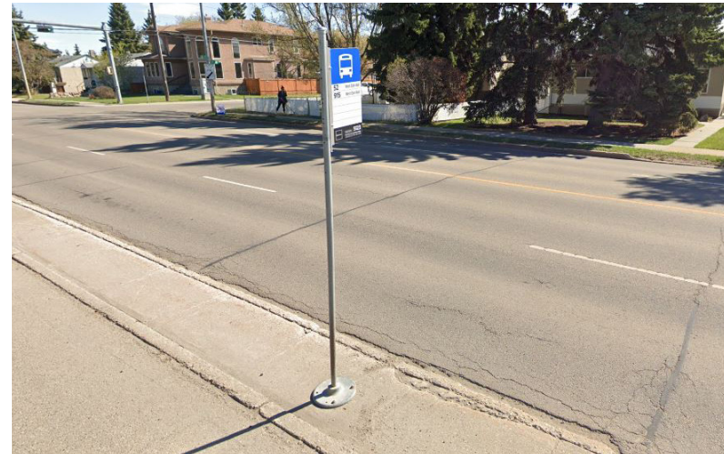
Bus stop without sidewalk access
