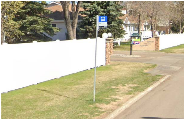
Bus stop without sidewalk access
