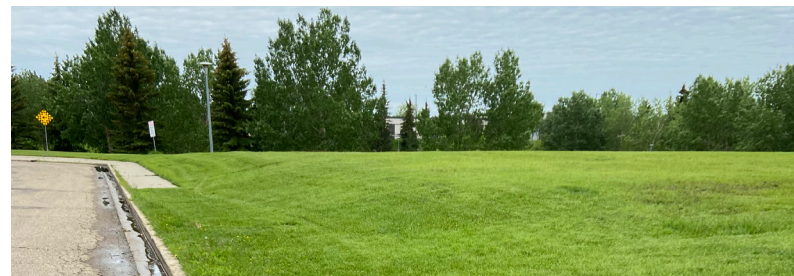
Missing sidewalk at Jack Horan Park
