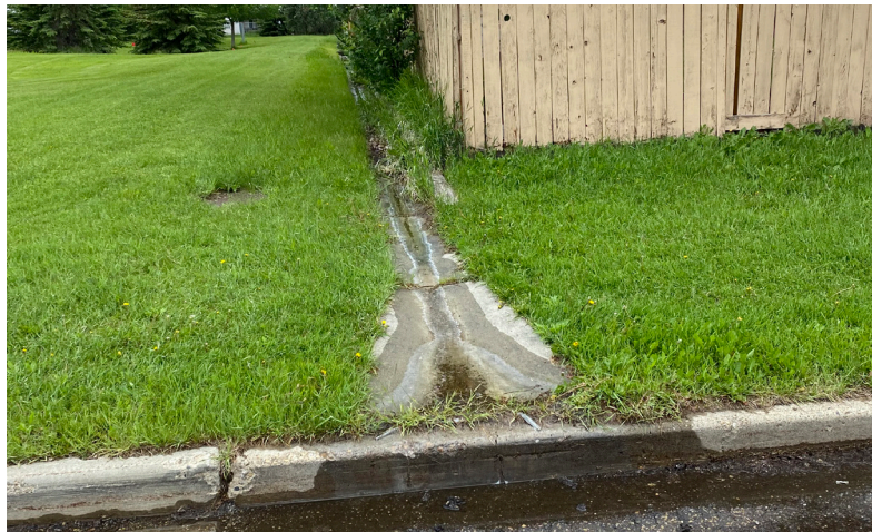
Drainage swale along fence located east of Jack Horan Park
