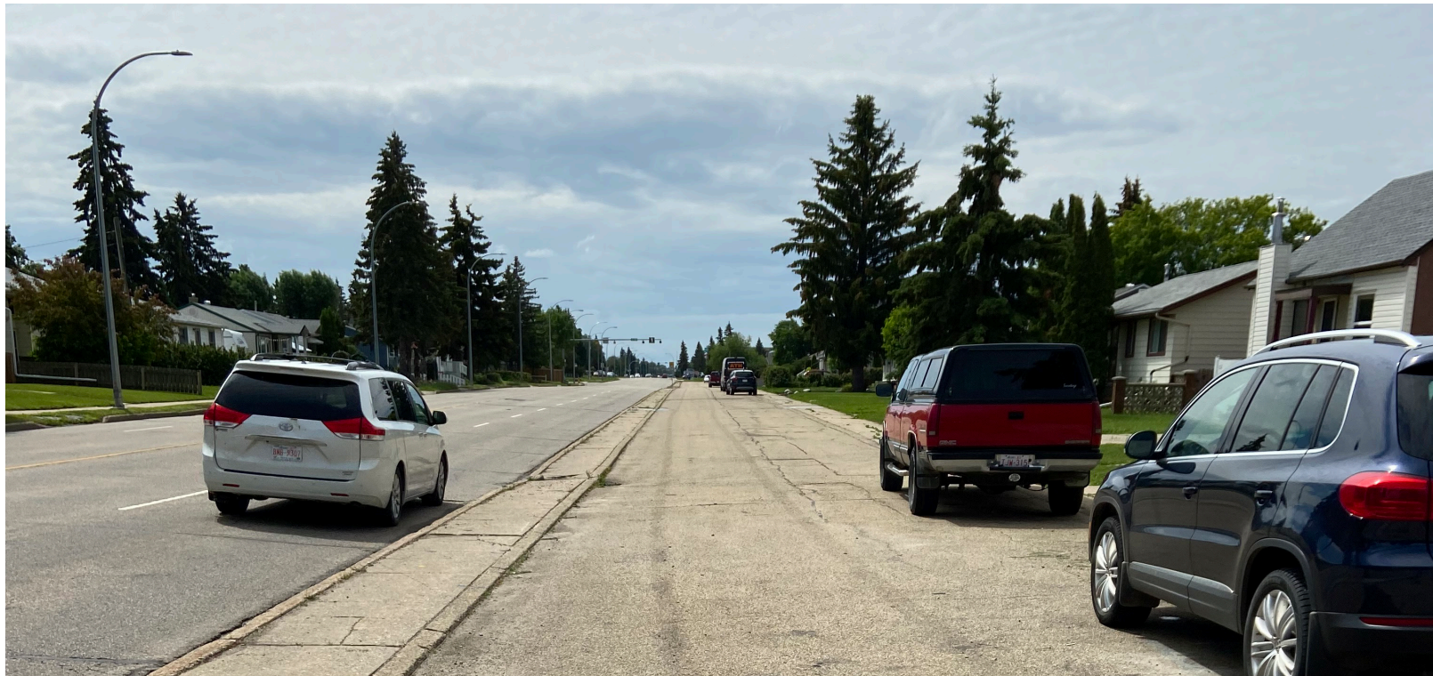
Eastern edge of West Glenwood at 163 Street
