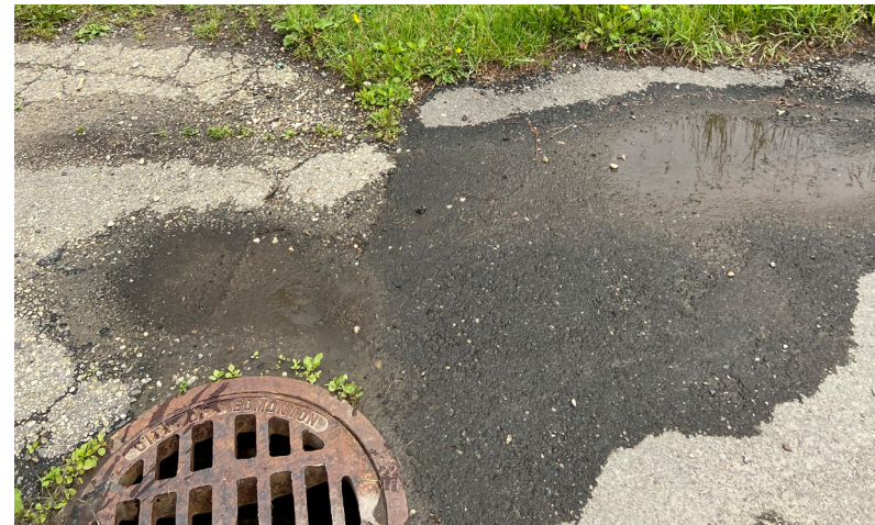
Manhole in West Glenwood
