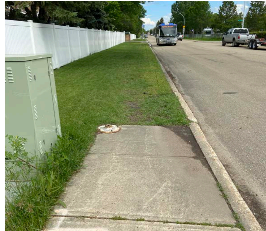
Discontinued sidewalk on 165 Street
