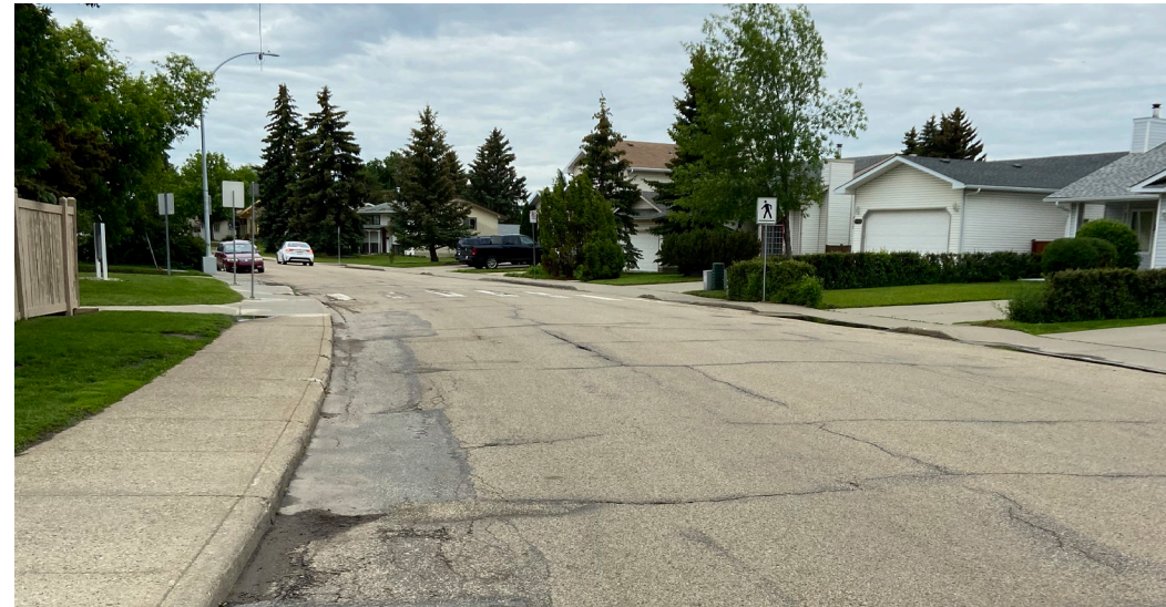
167 Street Collector Road in West Glenwood
