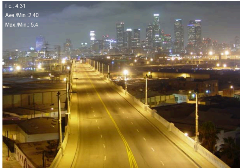
BEFORE (200 W HPS) 6th Street Bridge over Los Angeles River
