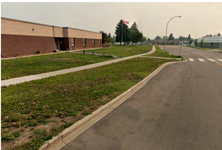
Photo of existing St. Maria Goretti School drop off
