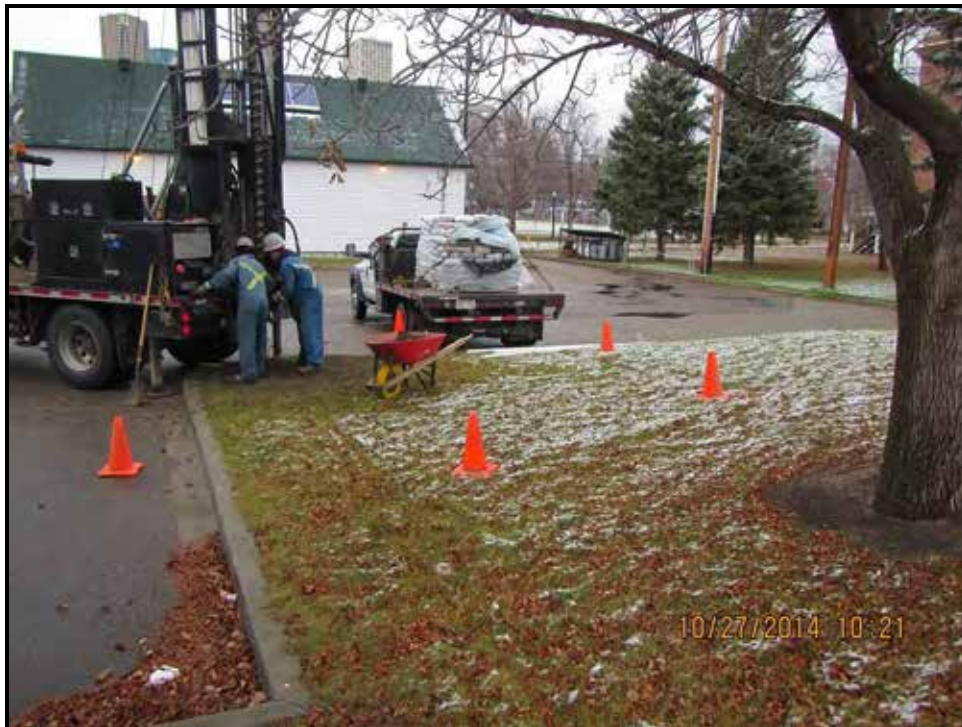
Photograph 4: Advancement of A5: 14-01 within Area 5 (background location), looking north.
