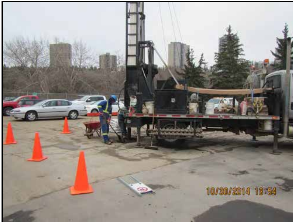
Photograph 3: Advancement of A3: 14-12 within Area 3, looking southeast.
