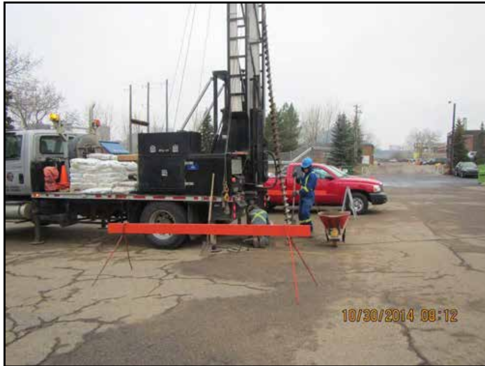
Photograph 1: Advancement of A3: 14-08 within Area 3, looking west.
