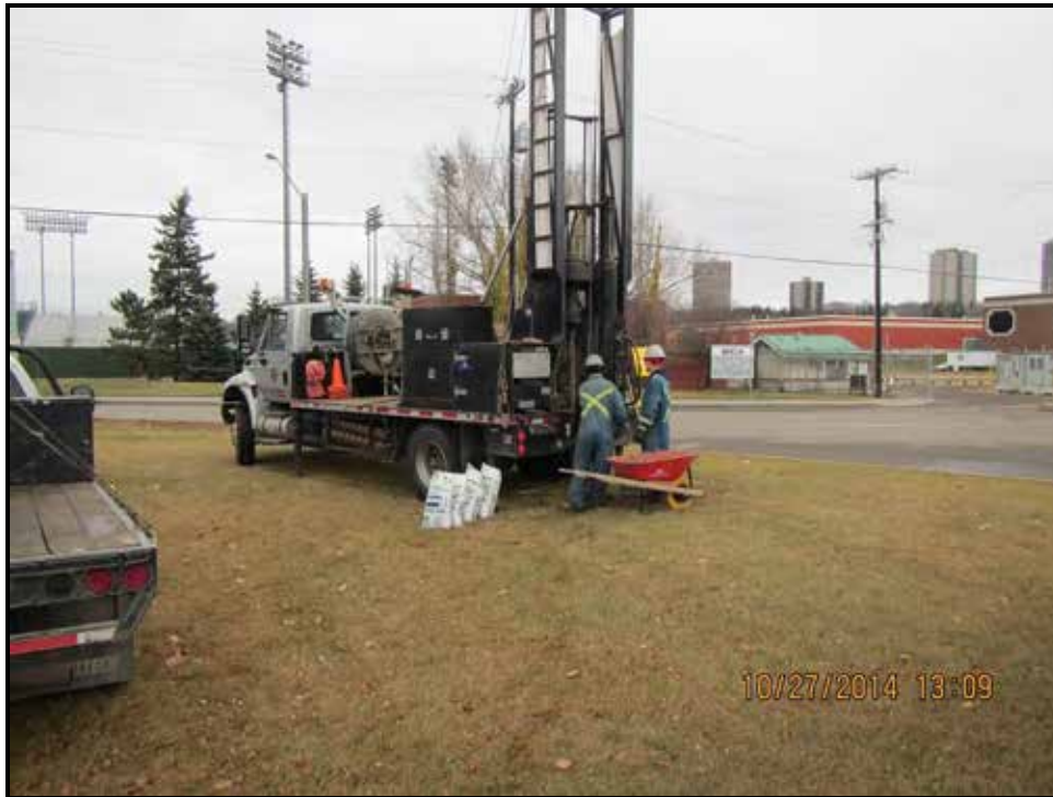
Photograph 5: Advancement of A5: 14-04 within Area 5, looking southeast.
