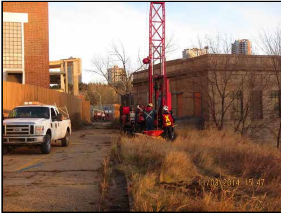
Photograph 7: Advancement of A6: 14-17 within Area 6, looking east toward Pump House #1.
