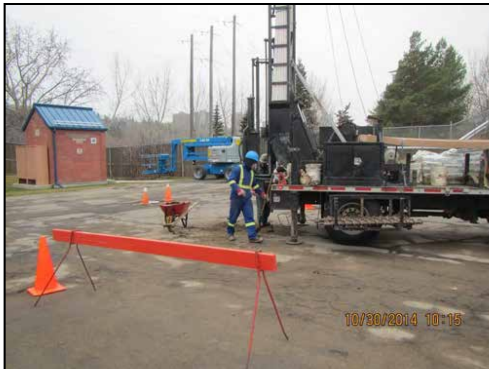
Photograph 2: Advancement of A3: 14-10 within Area 3, looking southwest.
