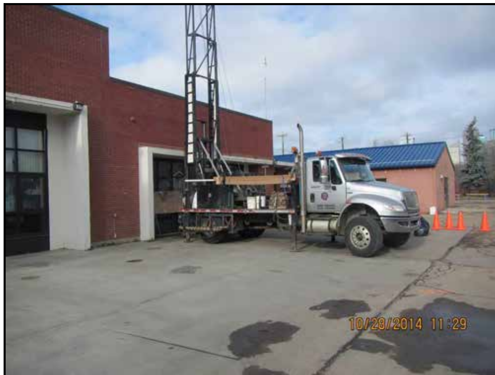
Photograph 10: Advancement of A7: 14-06 within Area 7, looking northwest.
