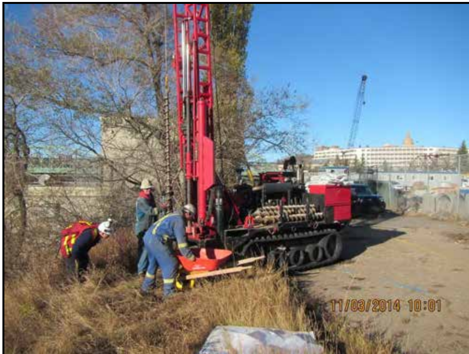
Photograph 6: Advancement of A6: 14-14 within Area 6, looking west toward Pump House #2.
