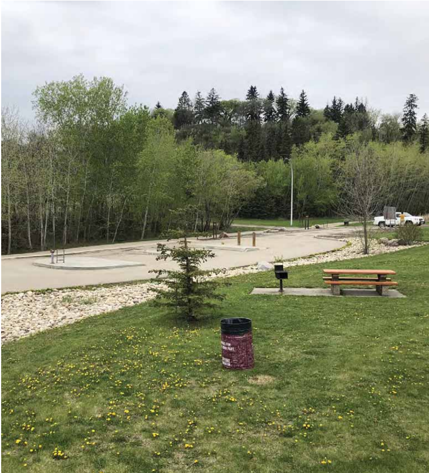
GROAT RAVINE UNDERGROUND TREATMENT
