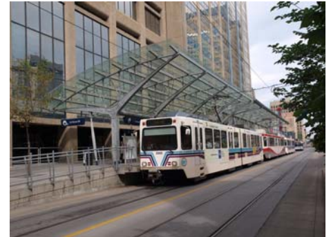
A high-floor LRT station integrated into a building in downtown Calgary, Alberta
