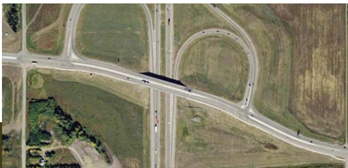
Anthony Henday Drive Ramps
