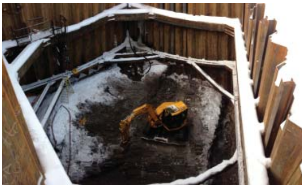
Excavation inside cofferdam
