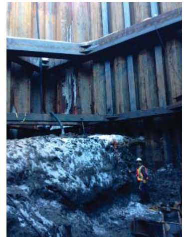
Worker inside cofferdam
